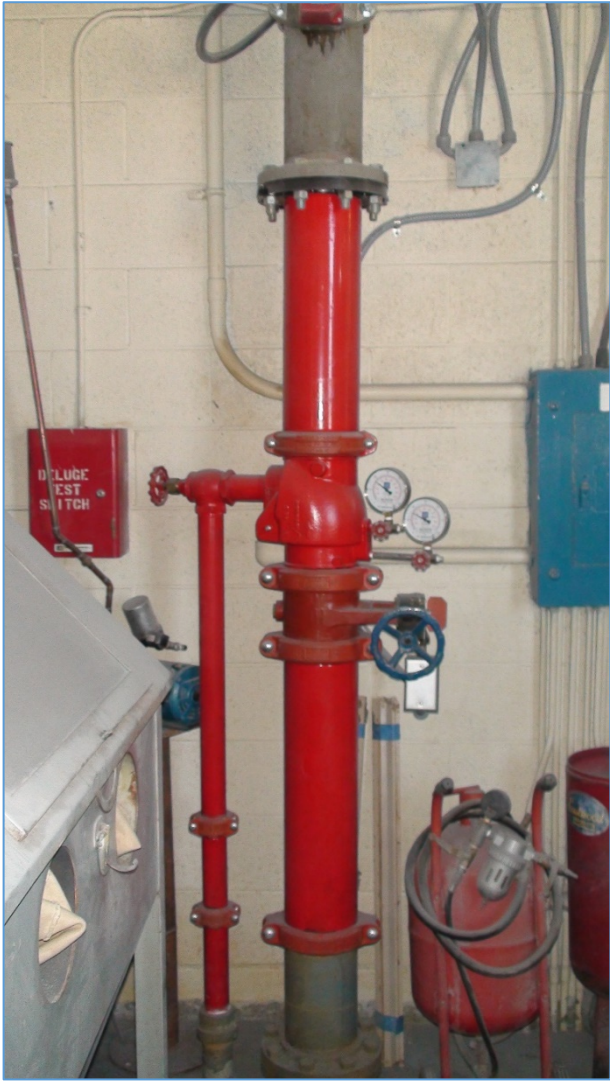
Hangar 510 (1959) wet pipe system
