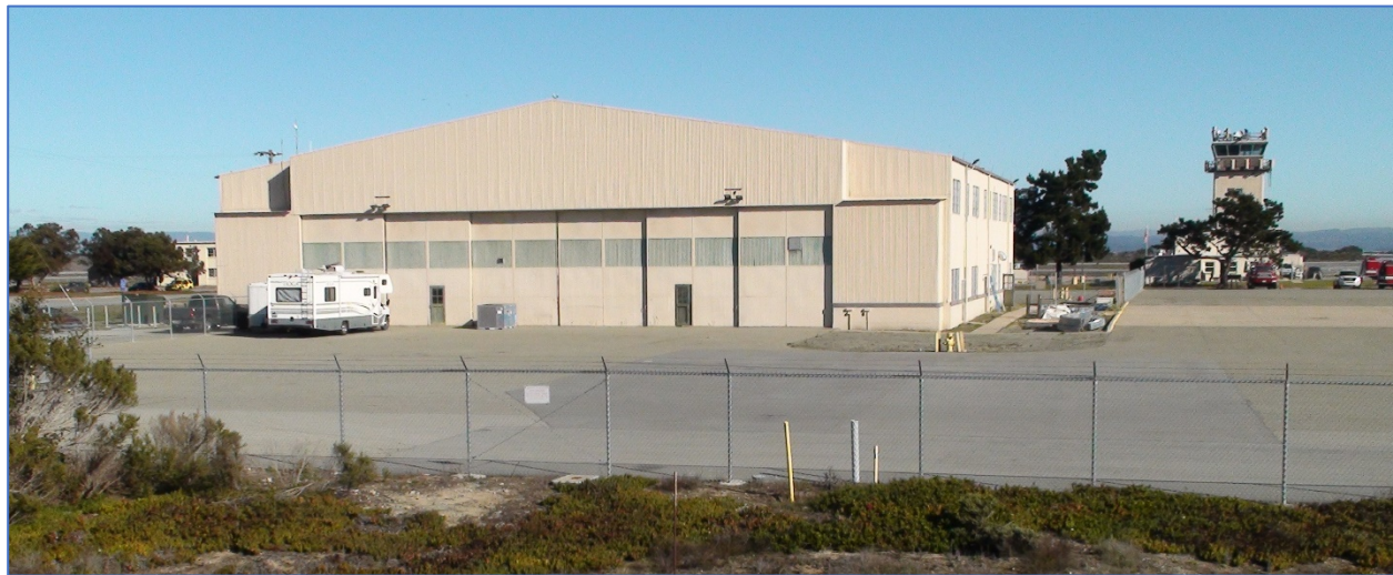
Photo 1: Building 510 and suspected infiltration basin (foreground), facing north
