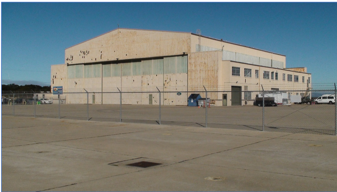
Photo 1: Exterior of Building 533, facing north
