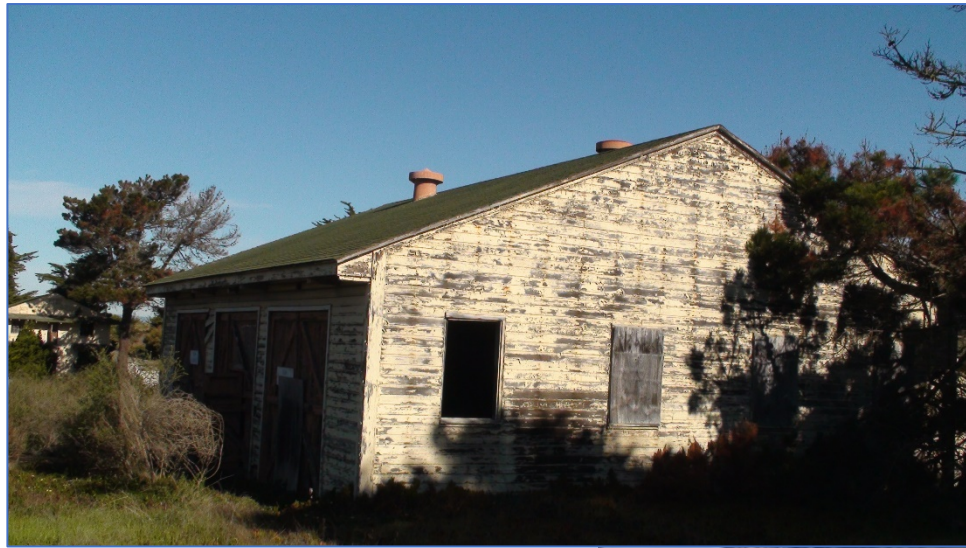
Photo 1: Exterior view of Building T-1820, facing north
