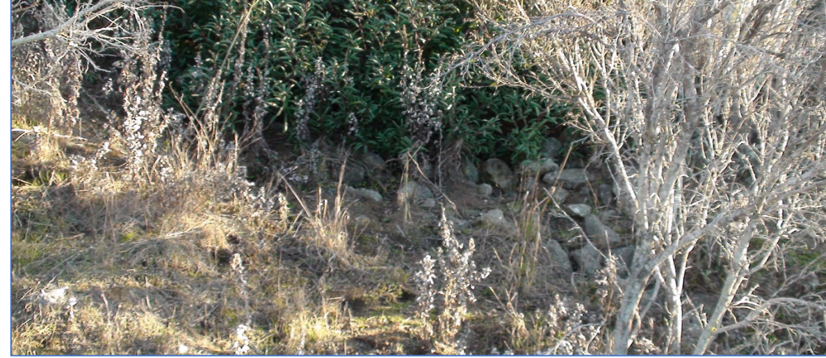
Photo 2: Stormwater outlet from Pete's Pond Extension to Pete's Pond, facing southeast
