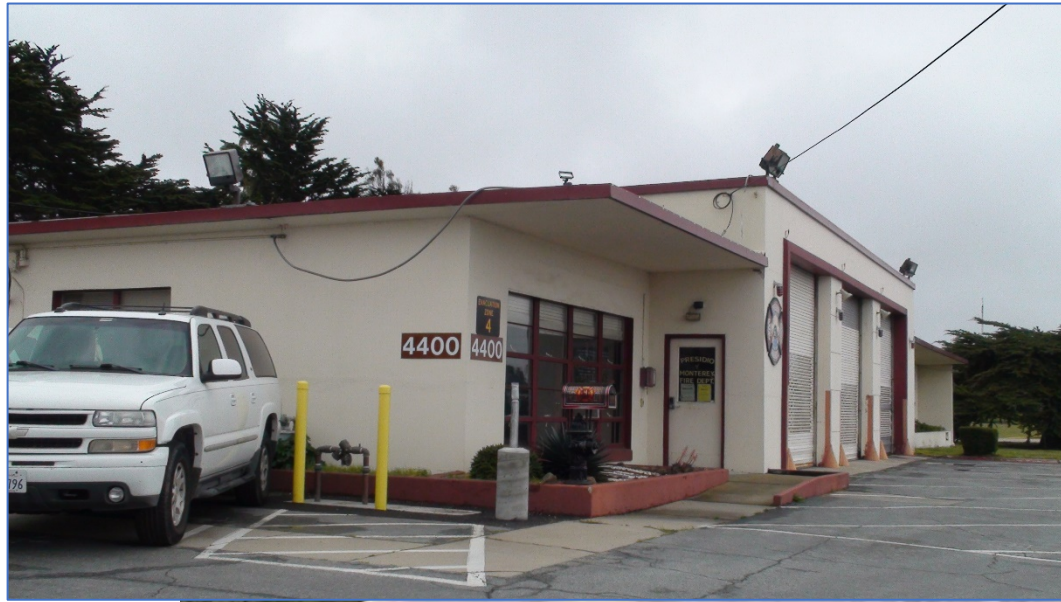
Photo 1: Building 4400 front, facing south
