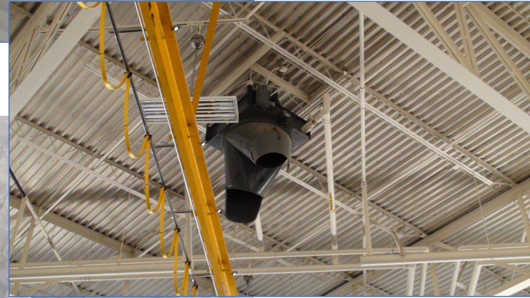
Photo 4: Hydronic heating system blower unit
