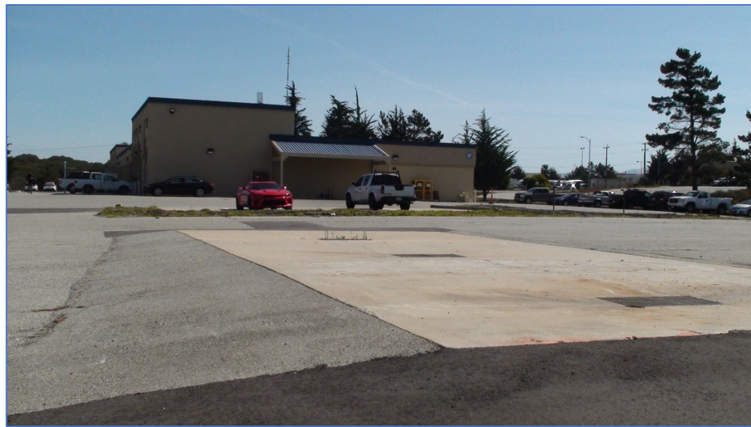
Photo 1: Building 4492 exterior and former wash rack, facing southeast
