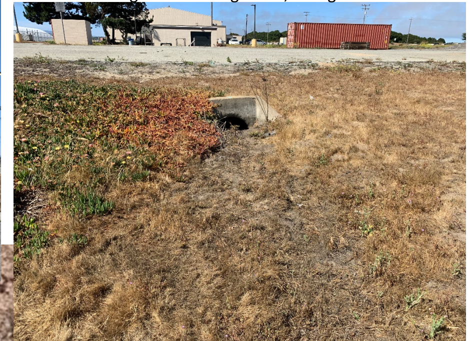
Photo 3: Discharge into drainage area, facing southwest
