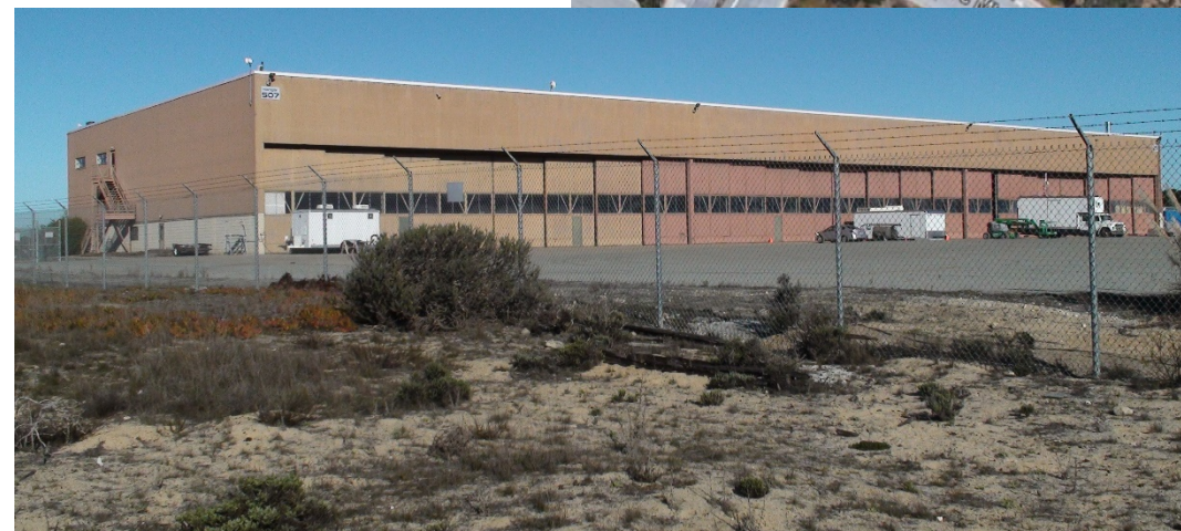
Photo 5: Eastern exterior of Building 507, facing northwest
