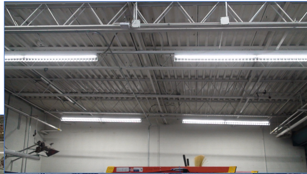
Photo 2: North garage area ceiling, facing west
