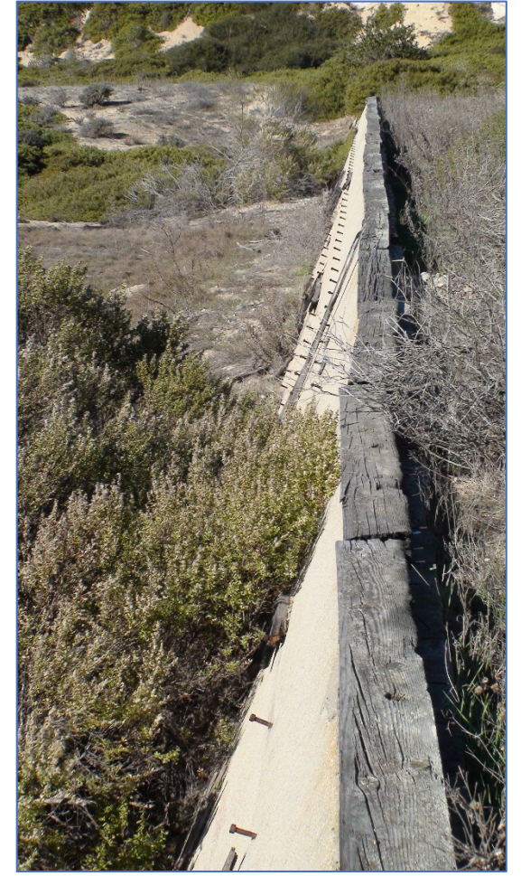
Photo 1: Retaining wall separating Range 40 (low-crawl area) and Range 40A, facing west
