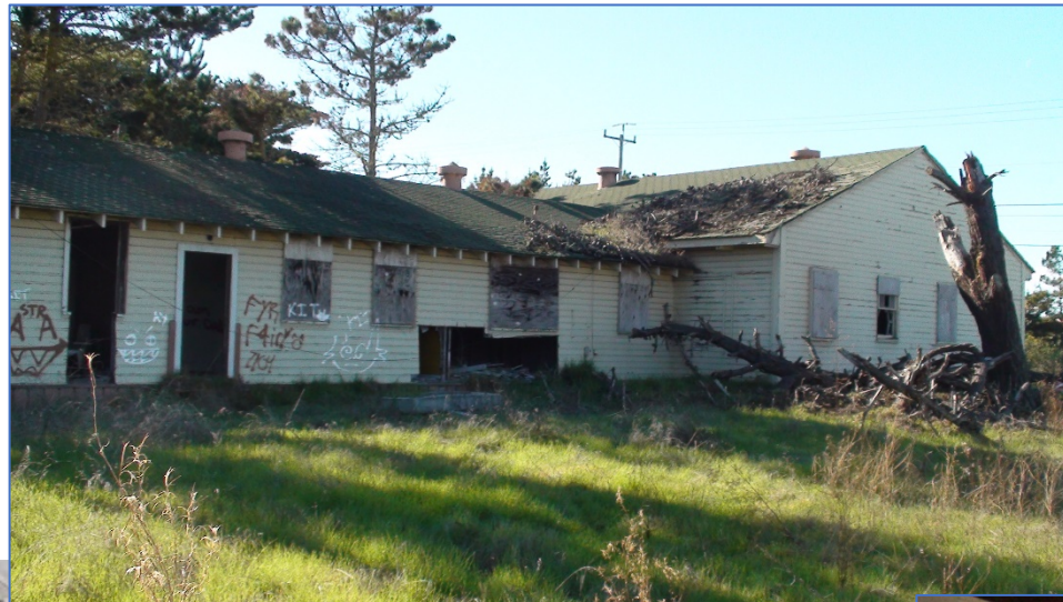
Photo 2: Exterior view of Building T-1820, facing southwest
