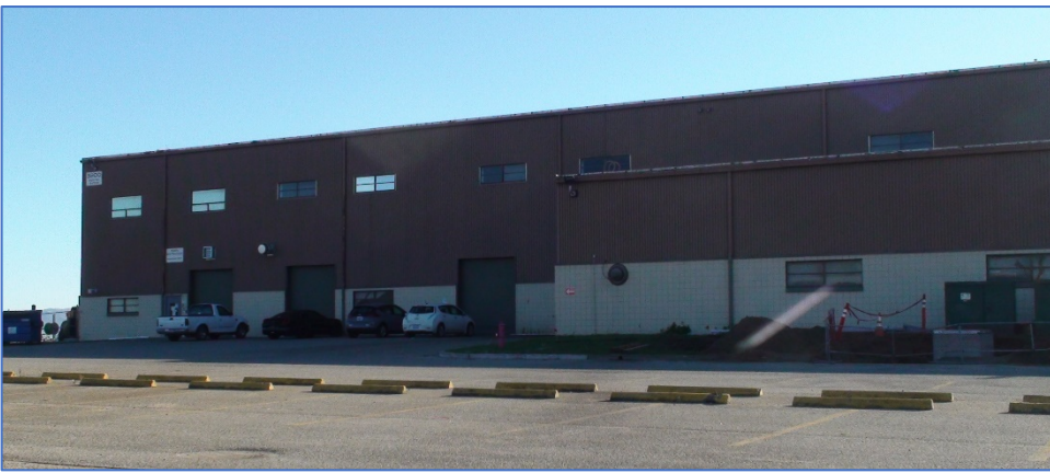
Photo 1: Western exterior of Building 507, facing east
