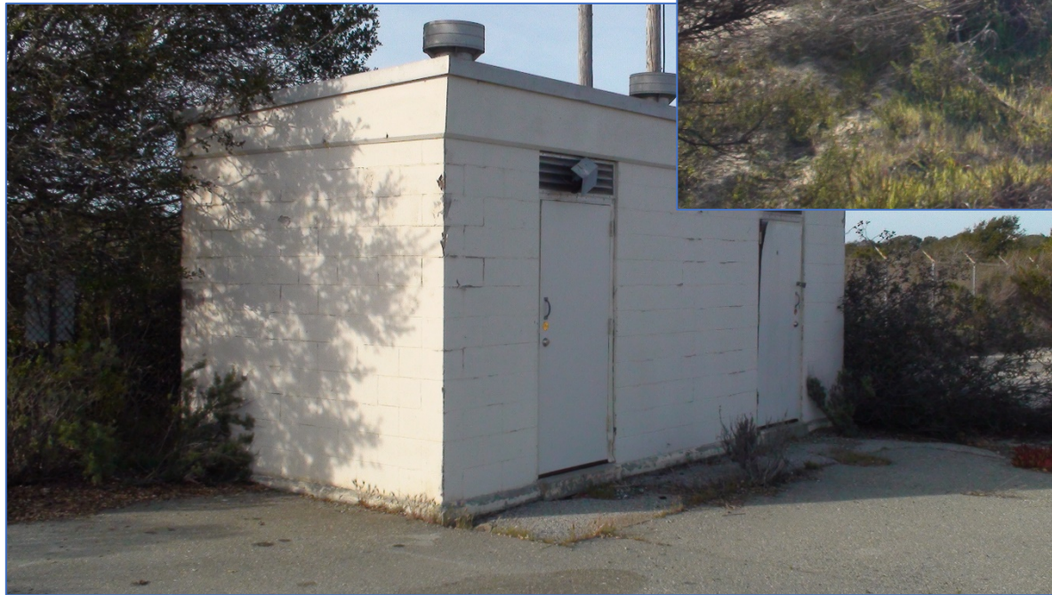
Photo 2: Building 502, facing north
