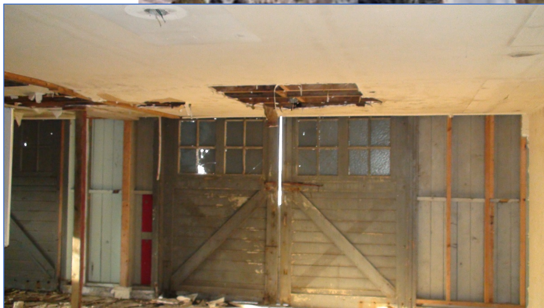
Photo 4: Interior view of drop ceiling blocking garage doors, facing west
