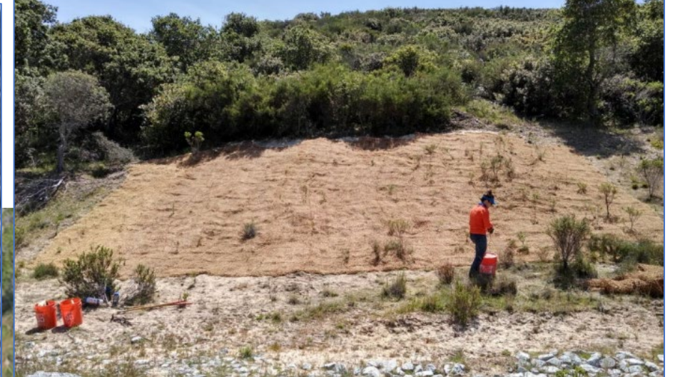
Photo 3: Installation of coir fabric at Range 34, facing east
