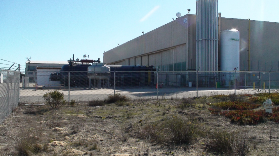
Photo 1: Building 527 and potential infiltration area, facing east
