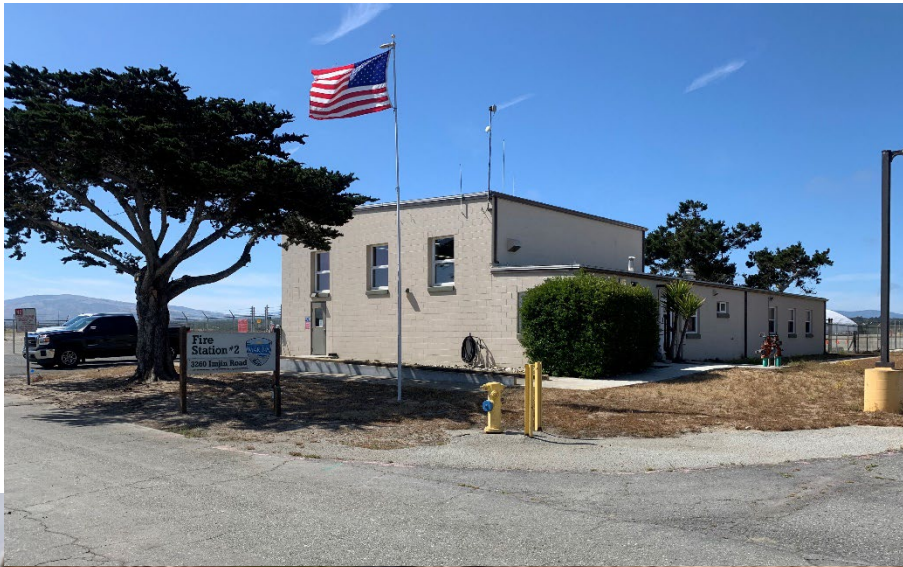
Photo 2: North side of station, facing south
