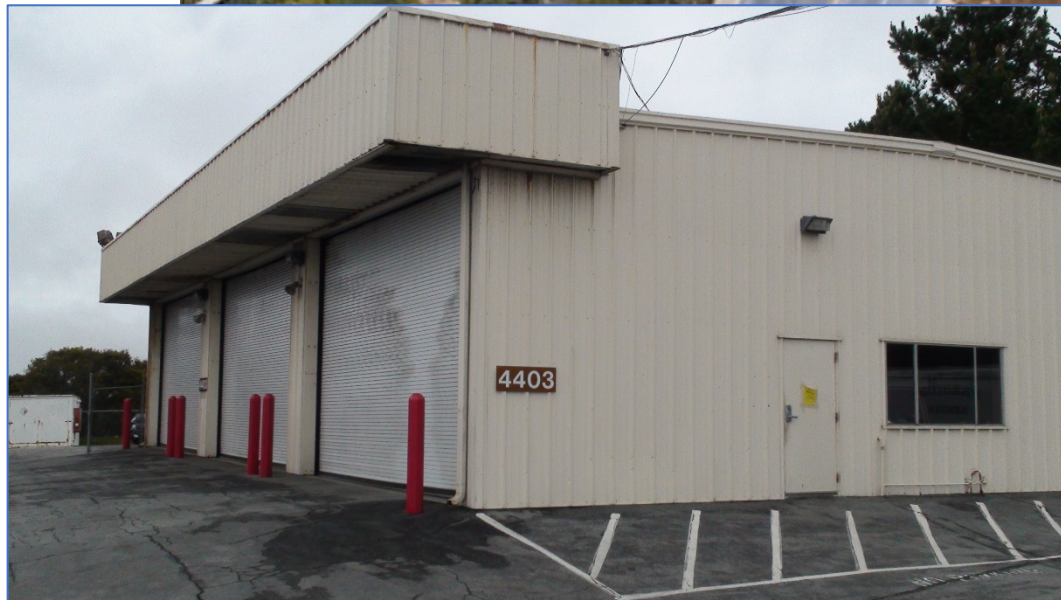
Photo 4: Building 4403, facing north
