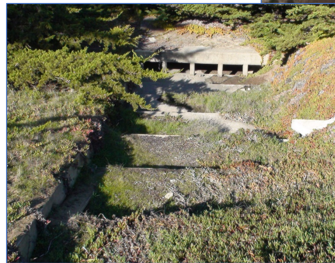
Photo 5: Storm drain inlet structure west of 2nd Avenue, facing west
