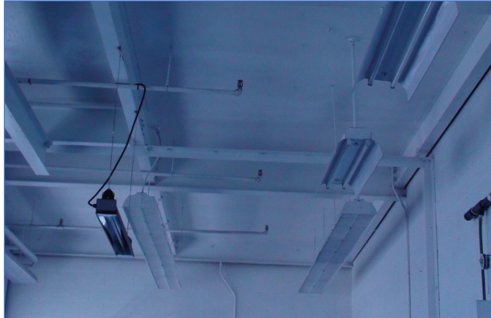
Photo 4: Workshop area wet-pipe sprinkler system
