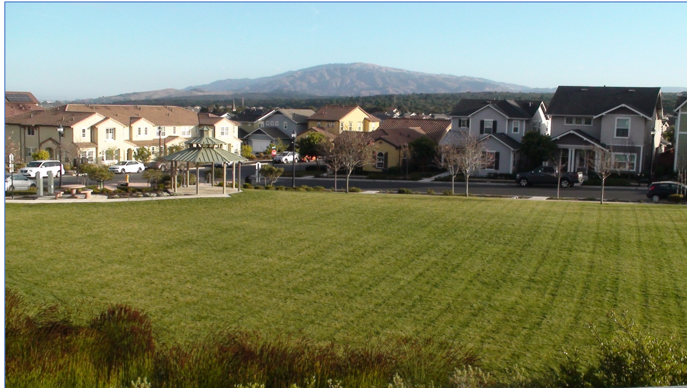
Photo 2: Overview of former East Garrison Sewage Treatment Plant area, facing southeast
