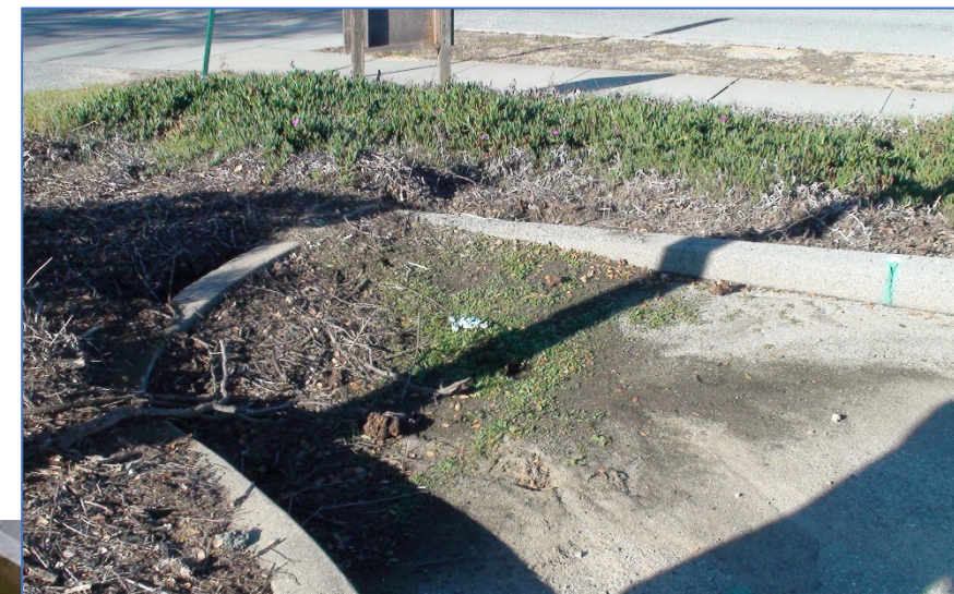
Photo 3: Southern storm drain inlet west of Building 507, facing west
