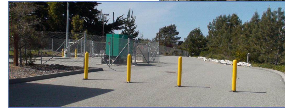
Photo 4: Sewage pump station area southwest of Promontory, facing west
