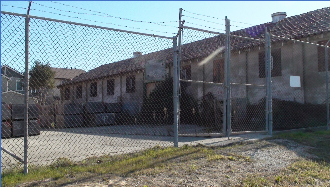
Photo 1: North side of Building T-111 and adjoining concrete-surfaced yard, facing south
