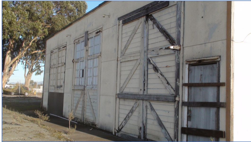
Photo 1: Exterior view of Building T-3280, facing east
