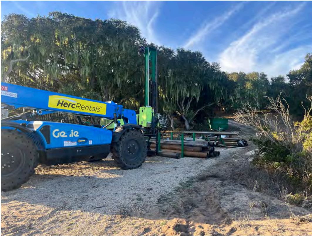
Photo 1. Well Installation Site MW-BW-97-A facing southwest, before installation.
