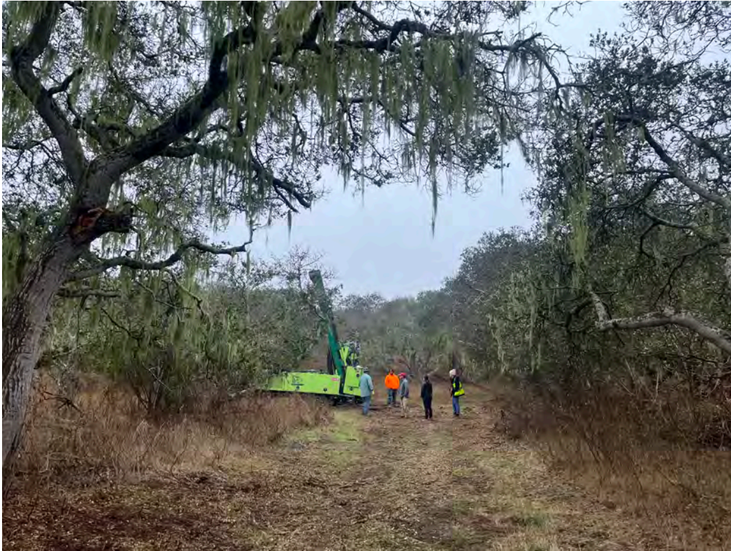
Photo 3. Well Installation Site MW-BW-96-A facing southwest, before installation.
