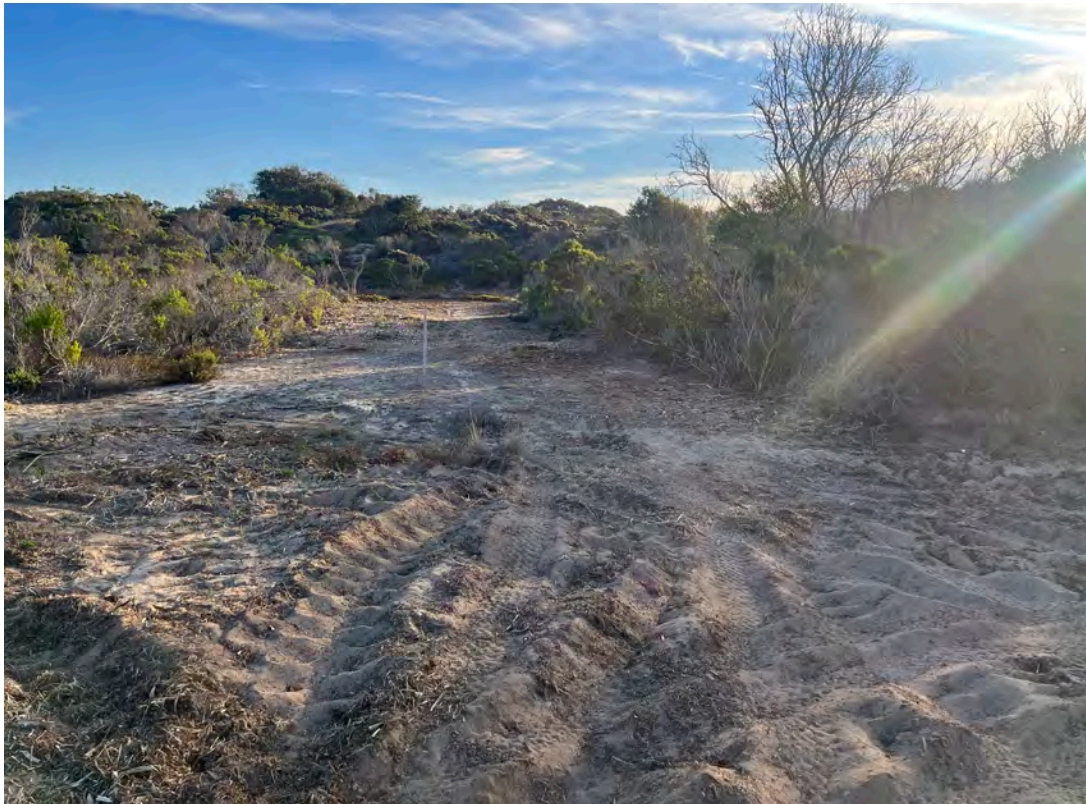
Photo 5. Soil Boring Location SB-FDA-01 facing east, before soil boring activities.
