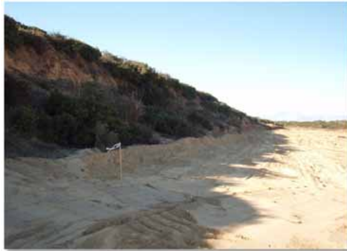
Photograph 3-3 – Range 47 SCA Sloped Escarpment
