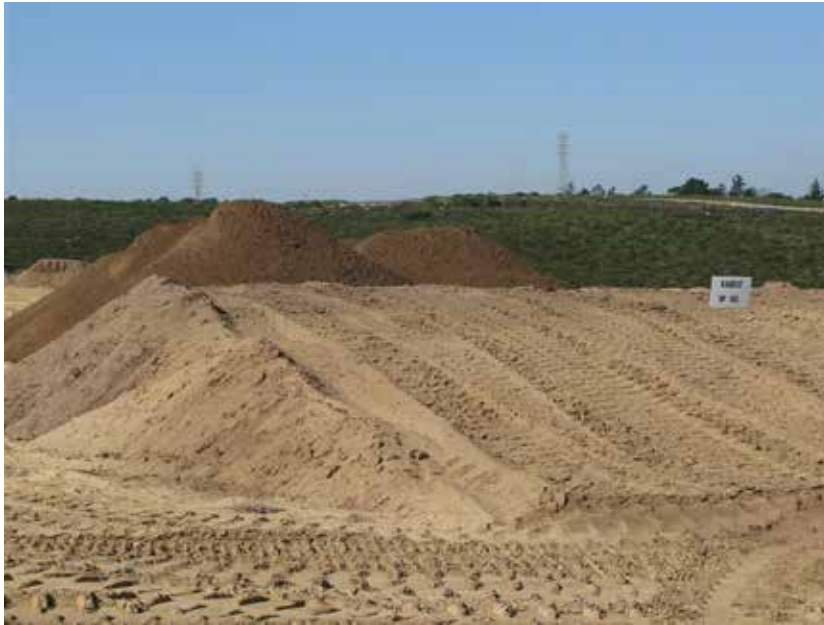
Photograph 1 – Interim Action Ranges MRA Development Parcel. Stockpiled topsoil from Range 47 prior to backfilling. 28 October 2012
