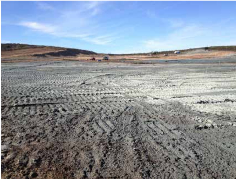
Photograph 13 – Interim Action Ranges MRA Range 47 Restoration Area Gray hydromulch application on soil surface for erosion control. 18 January 2013
