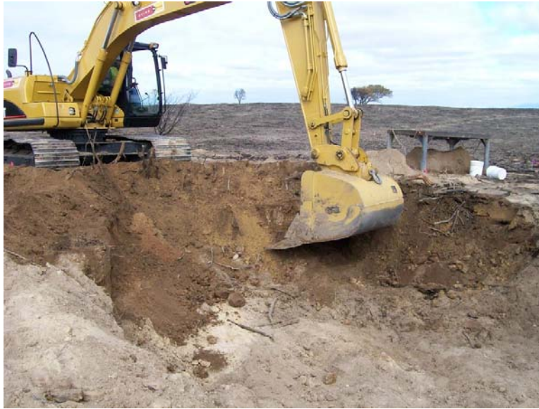
Photograph 13 Excavator at Pit
