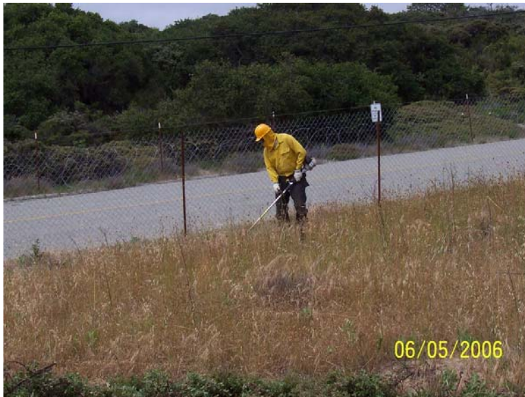
Photograph 4 Manual Vegetation Clearance
