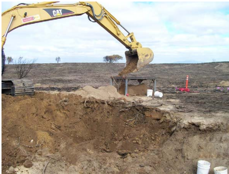
Photograph 14 Excavator Placing Spoils on Screen
