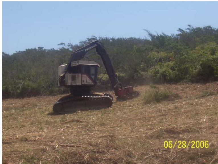
Photograph 1 Mechanical Vegetation Clearance
