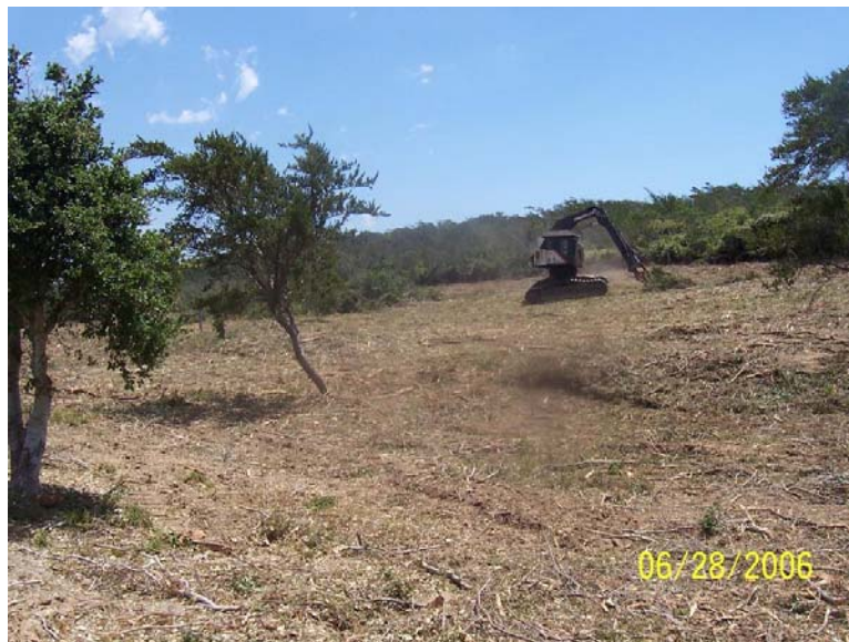
Photograph 2 Mechanical Vegetation Clearance
