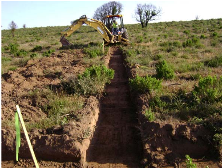
Photograph 16 Backhoe Completing Trench
