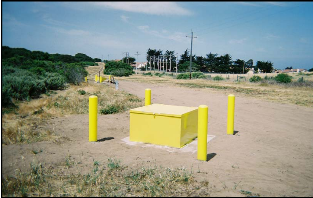
Photograph 1.2 – Typical new extraction well construction.
