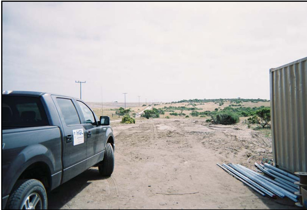
Photograph 1.3 – View of grassland area after clearing for infiltration trenches.
