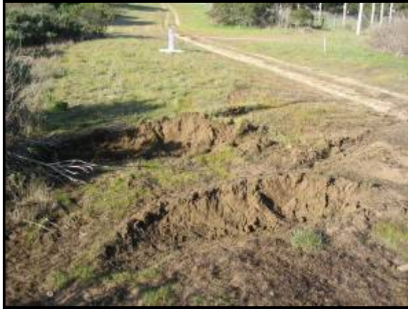
Photograph 3.1 – Tire ruts from construction equipment.
