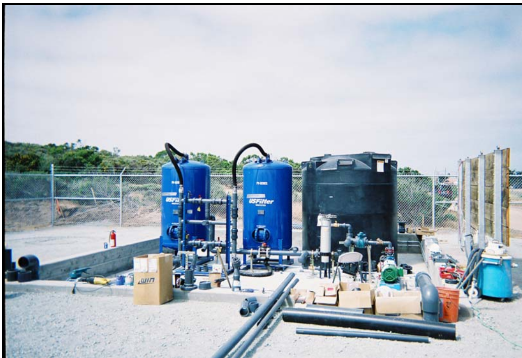
Photograph 1.4 – Construction of treatment plant facility.
