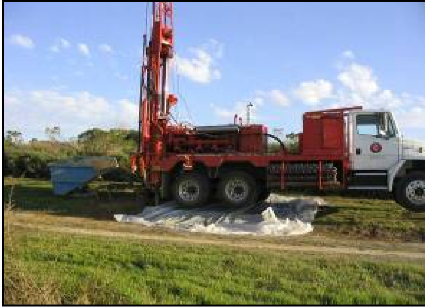
Photograph 1.8 – Typical spill containment technique used during drilling.
