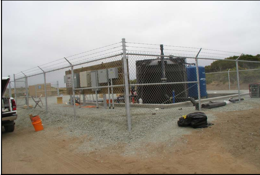
Photograph 1.5 – View of treatment plant facility looking west to east (roadway in the lower left foreground is the FONR northwest boundary road).
