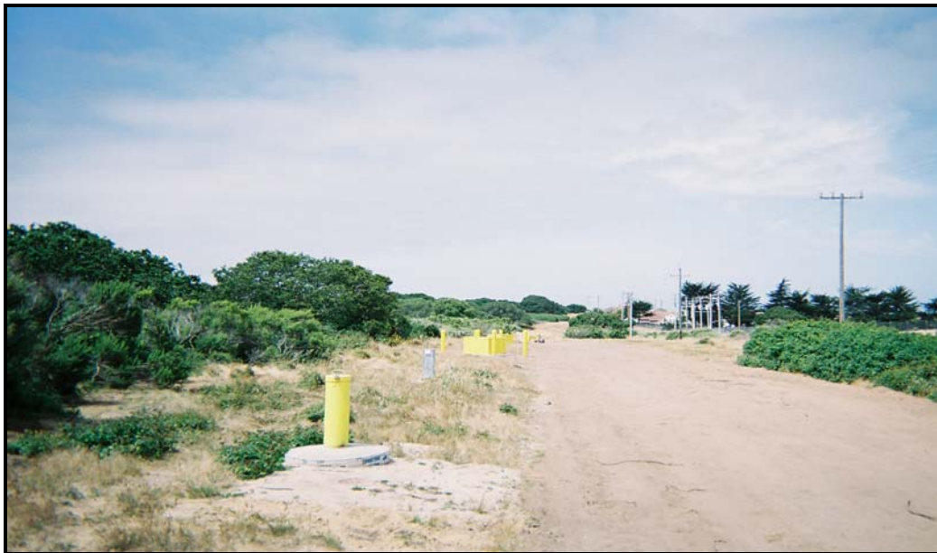
Photograph 1.1 – New wells constructed along FONR northwest boundary road.
