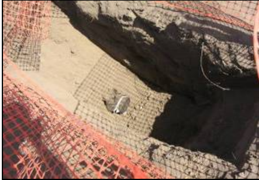
Photograph 1.7 – Example of covered pipe opening to prevent wildlife entrapment during 2006 HCPP construction.
