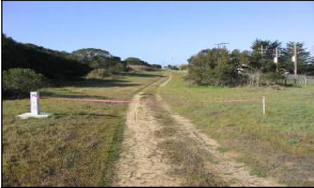
Photograph 1.6 – Boundary marker showing construction limit to avoid impact to rare plant populations during HCPP construction.
