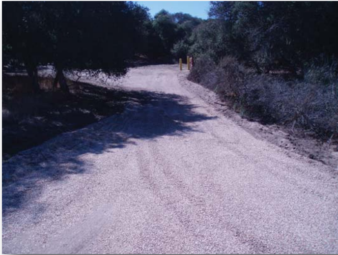
Photo 37. Gravel used to grade road along site 3 (looking Southwest).
