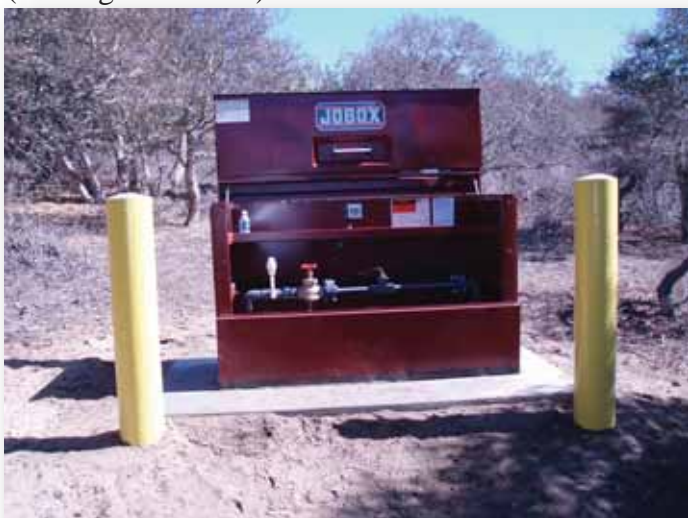
Photo 35. Completed well site MW-OU1-84-A.
