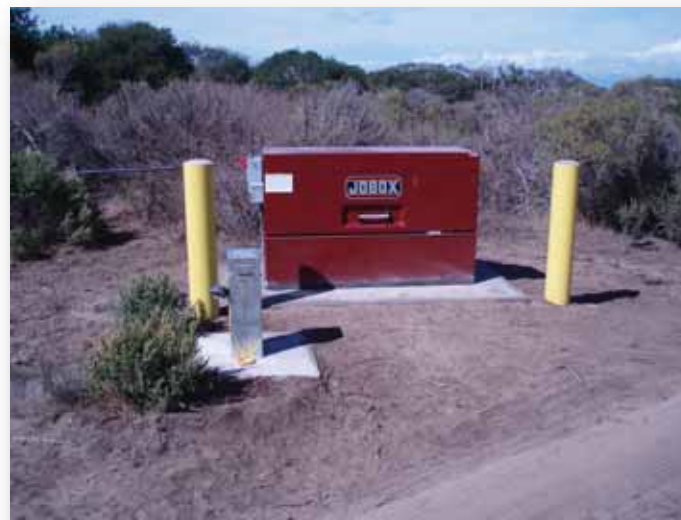
Photo 34. Completed well site MW-OU1-46-A.
