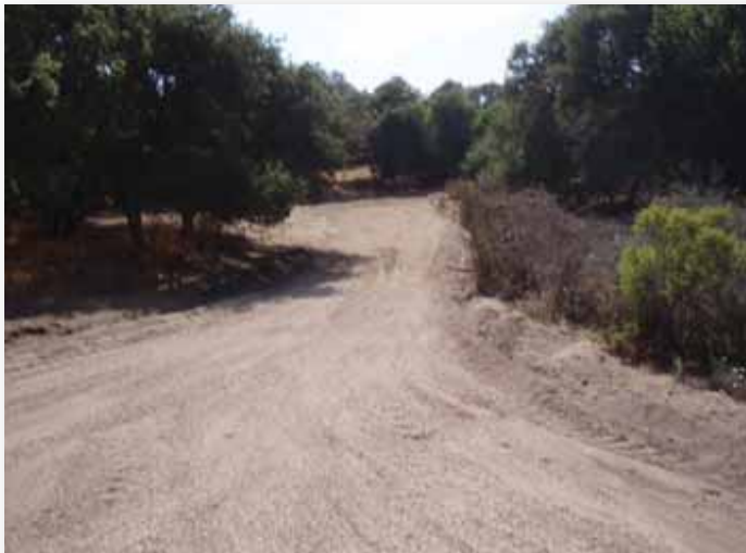
Photo 27. Regraded road along site three (looking Southwest).
