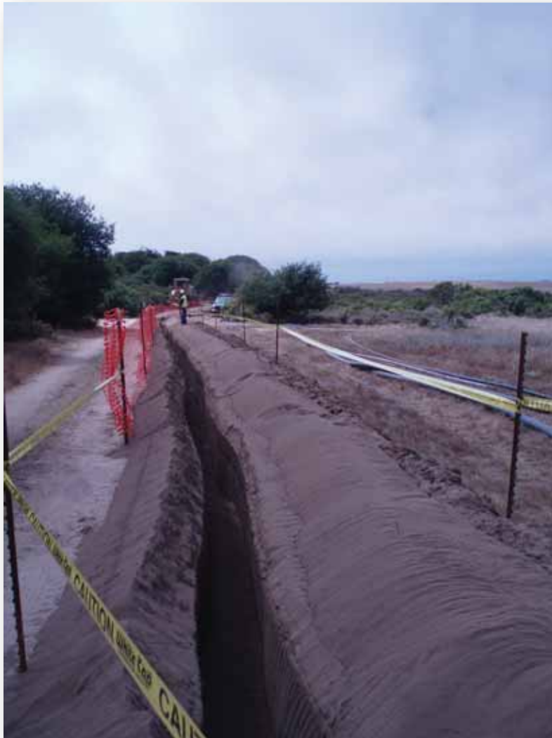
Photo 3. Trenches buffered with caution tape and fence (looking Northwest).
