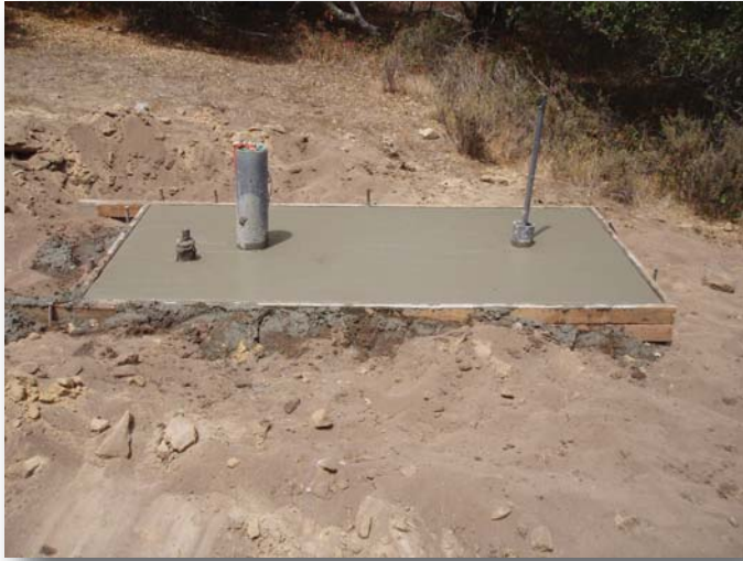
Photo 13. Concrete poured at well location EW-OU1-71-A.
