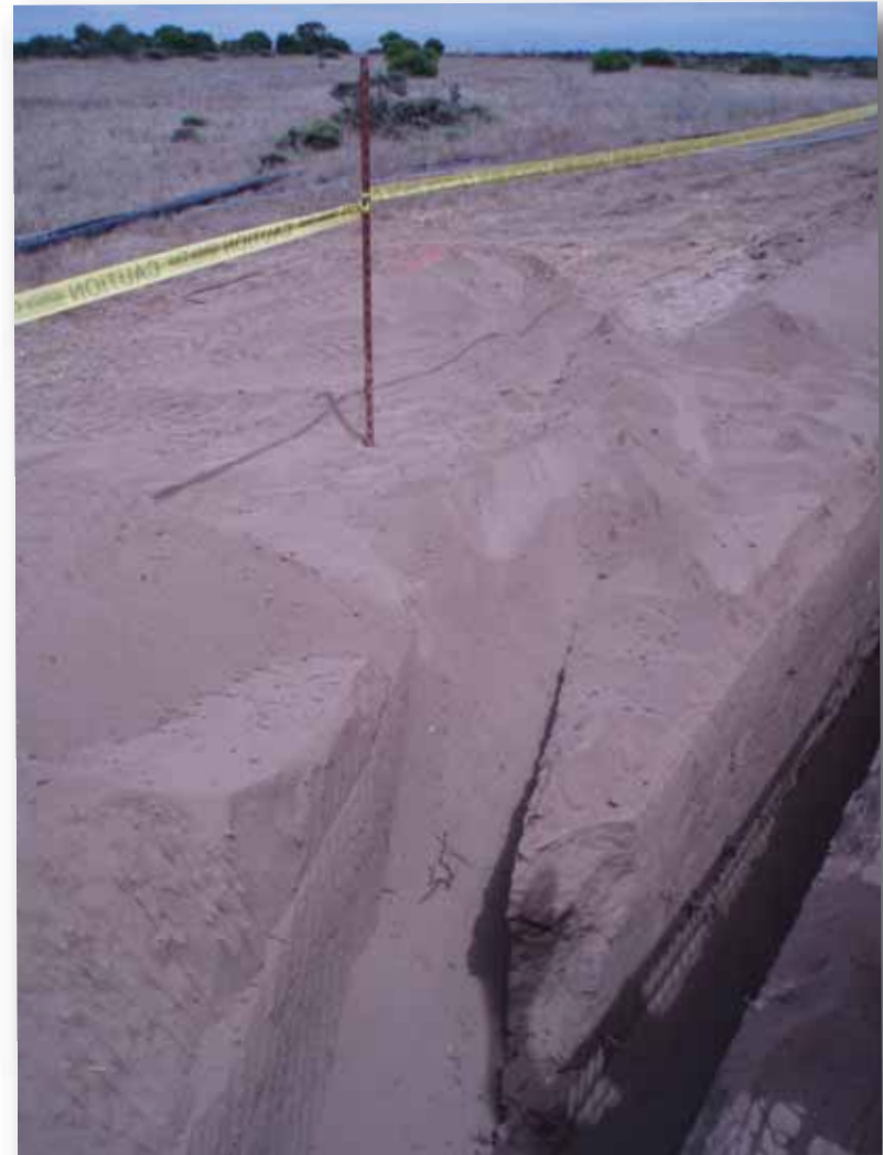
Photo 2. Close up of a dirt ramp (looking Southeast).
