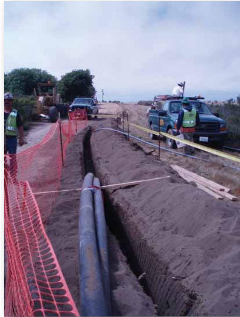
Photo 4. Pipe installation (looking Northwest).
