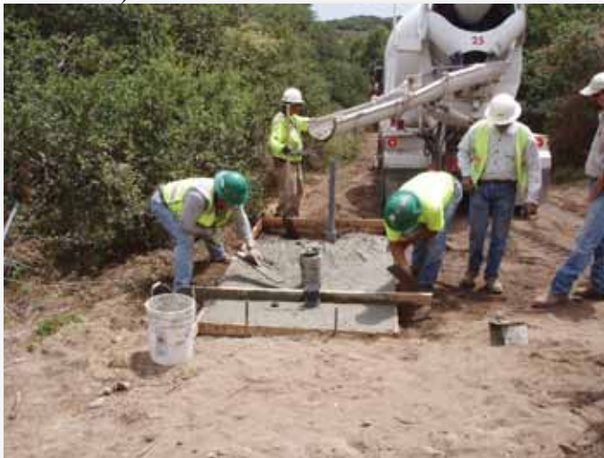
Photo 11. Pouring concrete at well location MW-OU1-85-A.
