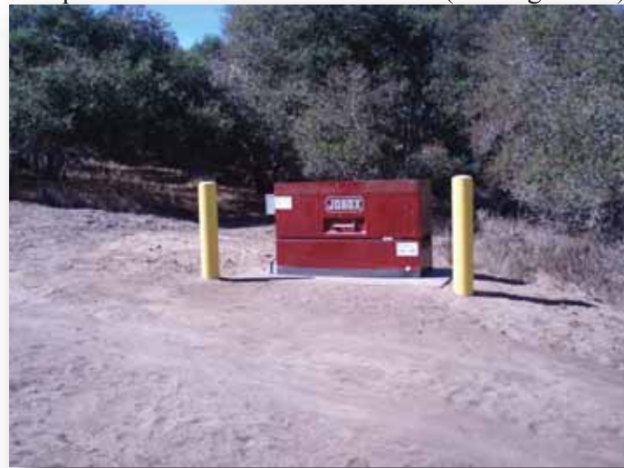
Photo 32. Completed well site EW-OU1-71-A.
