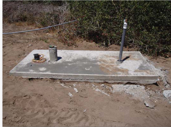
Photo 14. Electrical work at well location MW-OU1-85-A.
