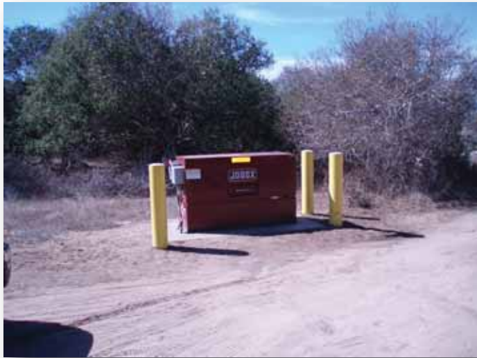
Photo 31. Completed well site MW-OU1-87-A.
