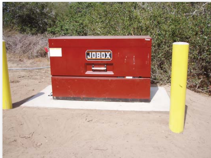
Photo 24. Spilled concrete cleaned up at well MW-OU1-85-A.
