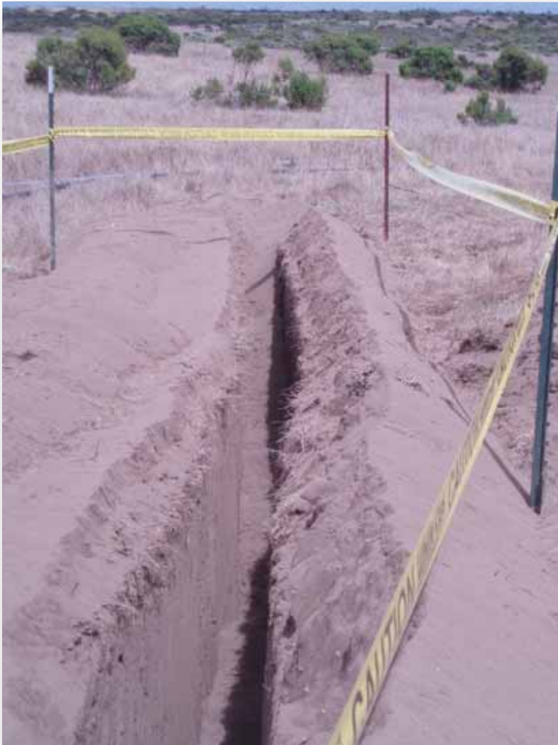
Photo 1. Trench with dirt ramp (looking East).
