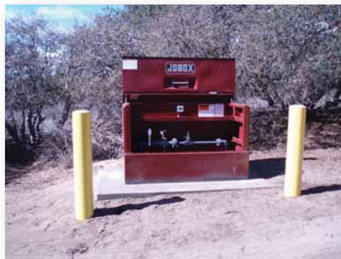
Photo 36. Completed well site IW-OU1-74-A.
