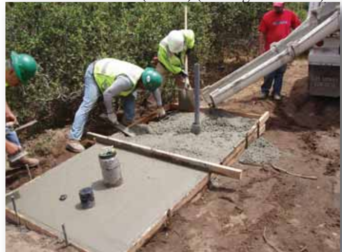
Photo 12. Pouring concrete at well location MW-OU1-85-A.
