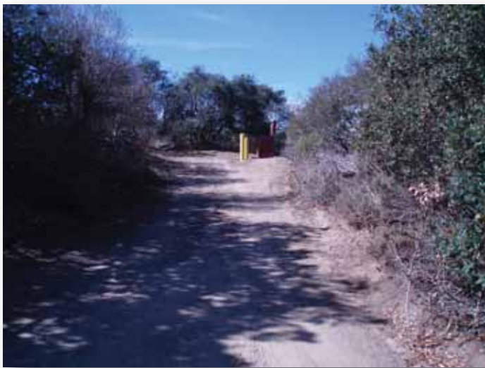
Photo 33. Completed well site MW-OU1-85-A (looking Northwest).
