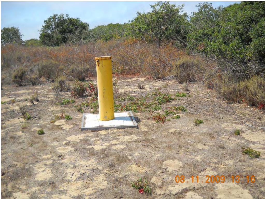
WCS# 06A ps12a EW-OU1-53A Post-Treatment 11 August 2009
