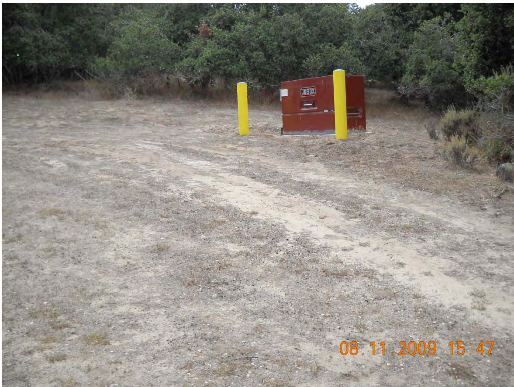
WCS# 11A ps44a EW-OU1-71A Post-Treatment 11 August 2009
