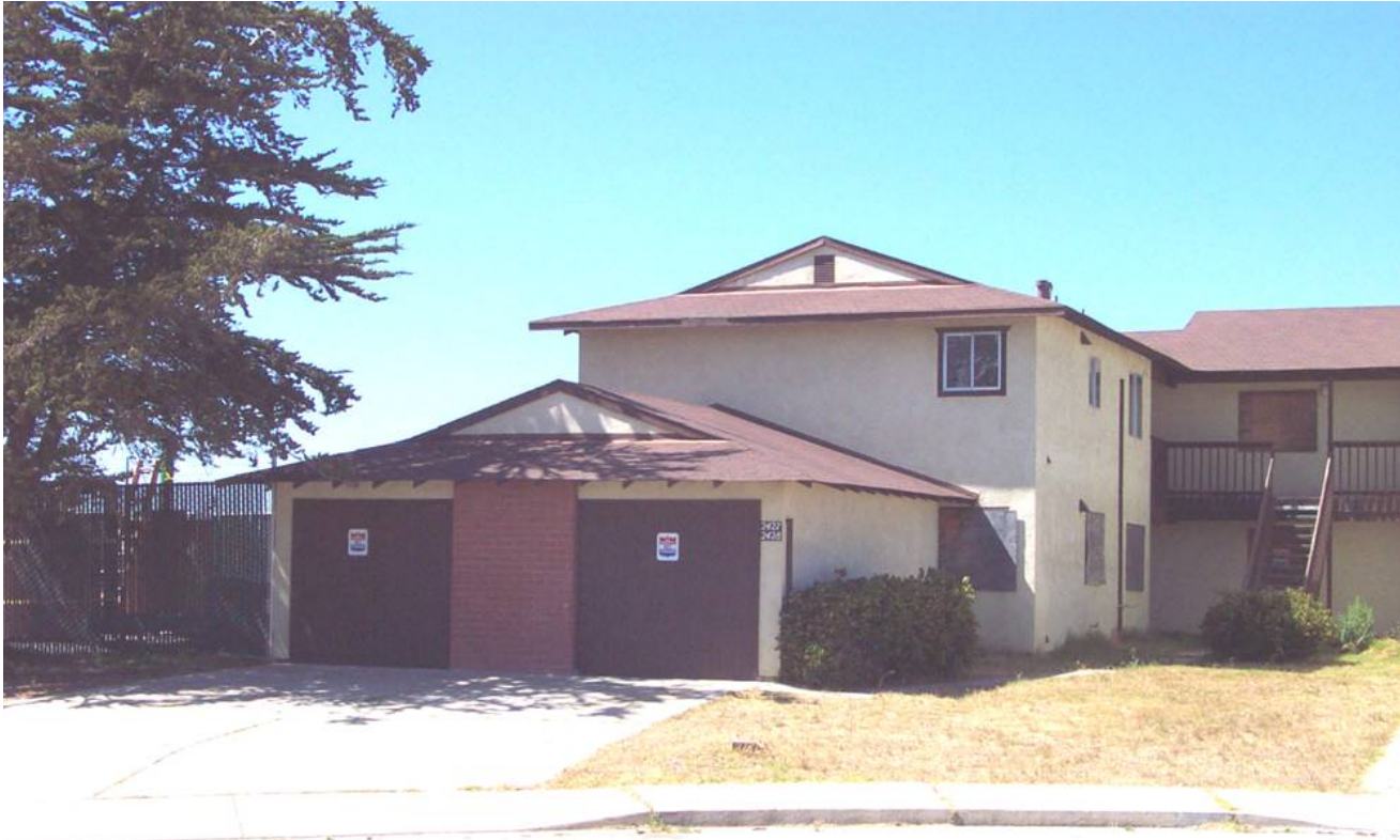
Photograph 1-1 Lexington Court Building
