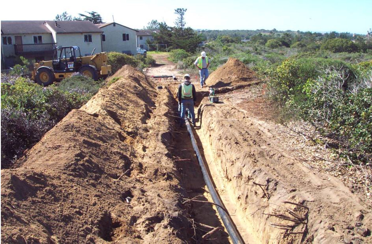
Photograph 2-2 Pipeline Installation
