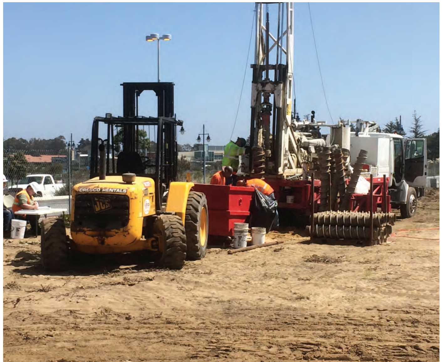
Drill rig at the Pilot Study location
