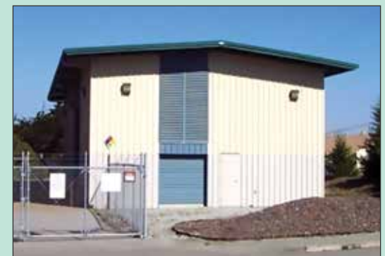
Sites 2/12 treatment plant
