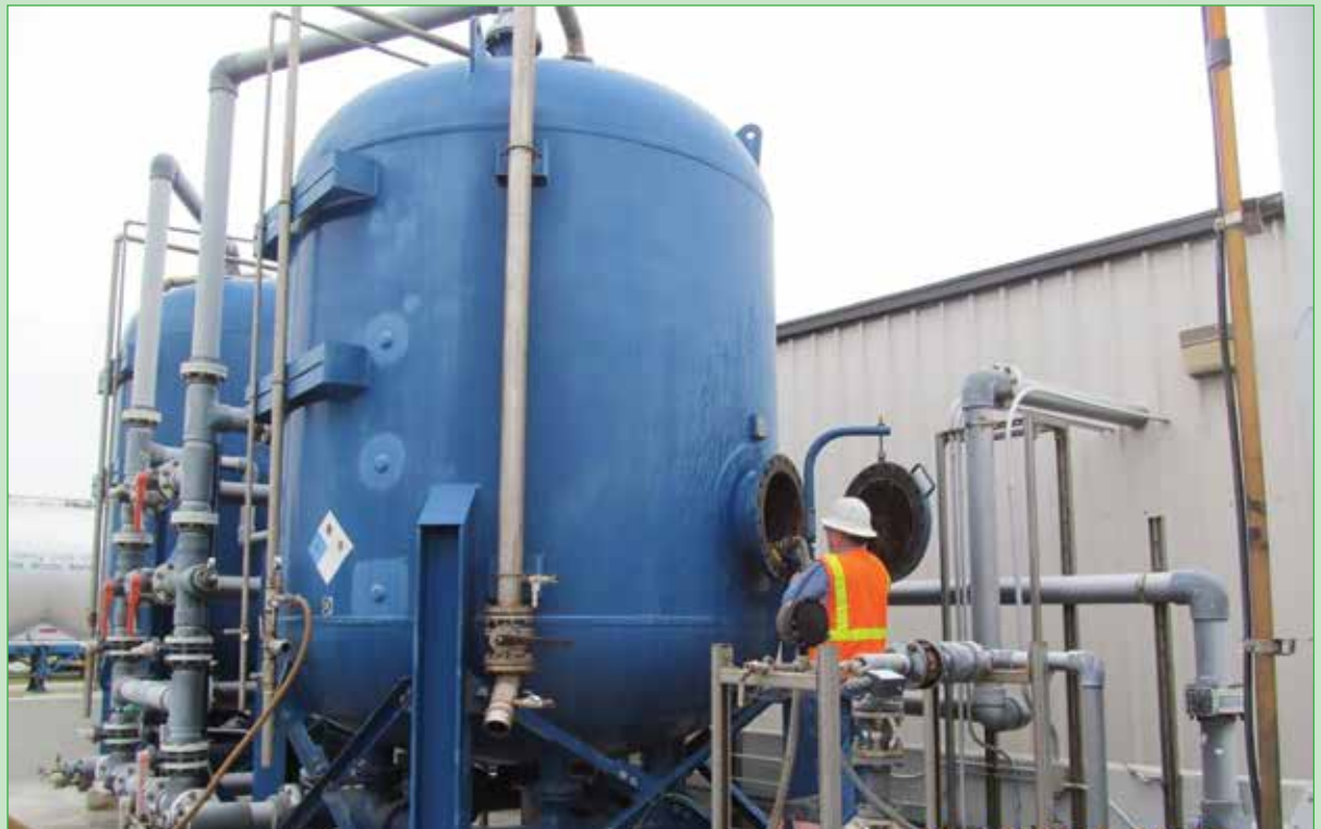
Photos show (above) removal of spent carbon from tanks and (below) installation of replacement, fresh carbon from tanker truck.
