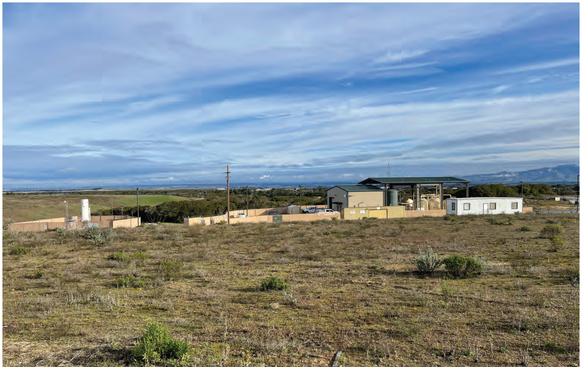
Operable Unit 2 Groundwater Treatment Plant (see page 4 for more information)
