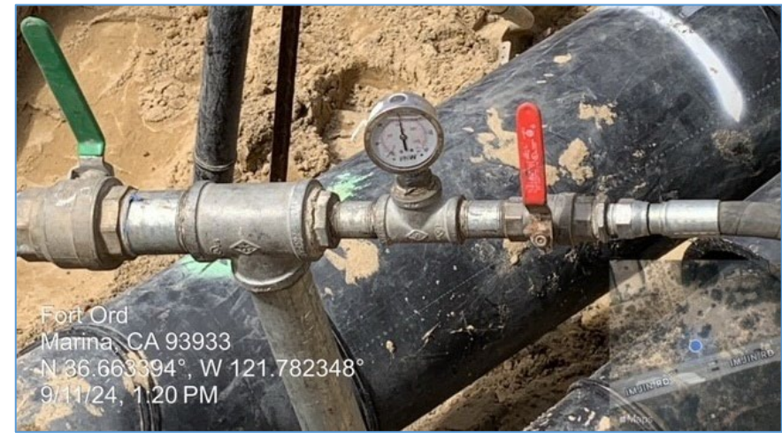
Pressure testing assembly
