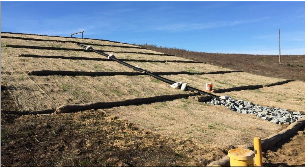
Area F vegetative cover erosion repairs
