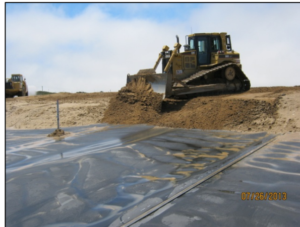
Placing vegetative cover soil
