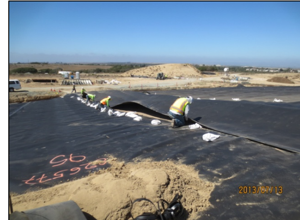
Joining geomembrane seams
