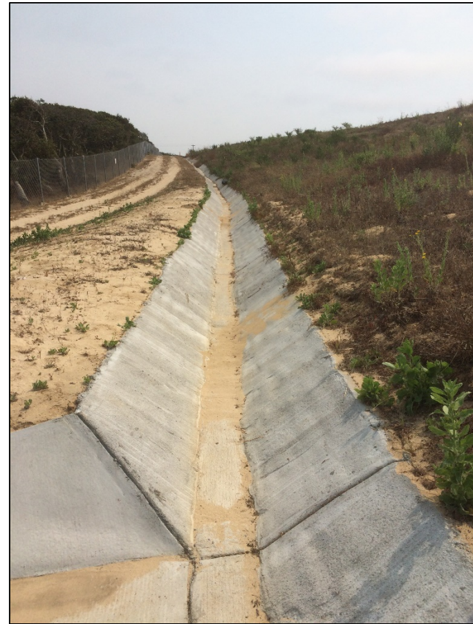
Area E concrete lined drainage ditch
