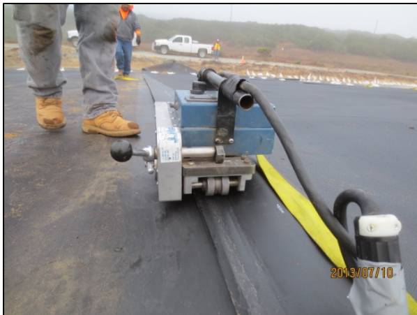
Welding geomembrane seams
