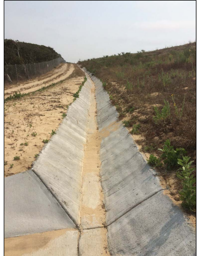
Area E concrete lined drainage ditch
