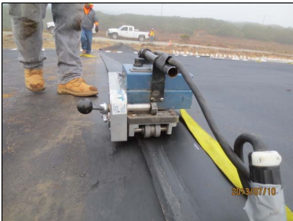
Welding geomembrane seams
