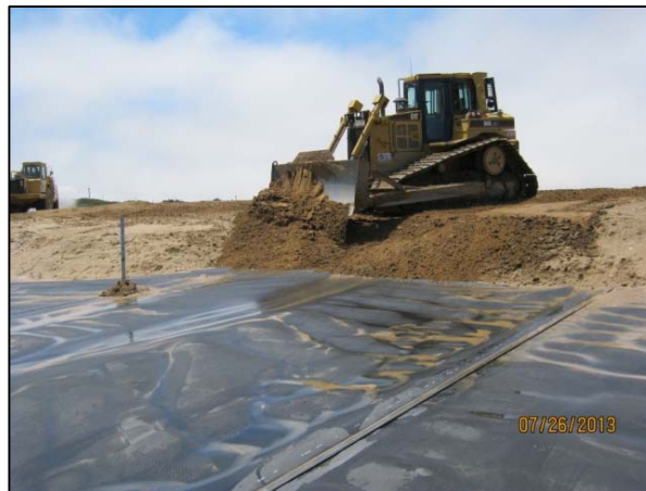
Placing vegetative cover soil
