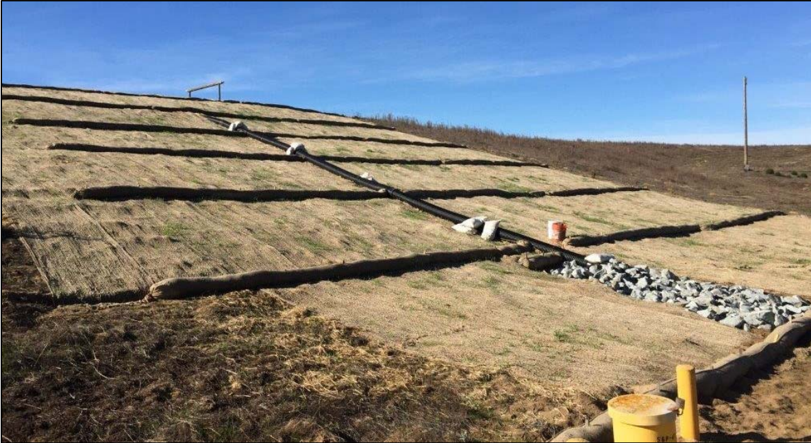
Area F vegetative cover erosion repairs
