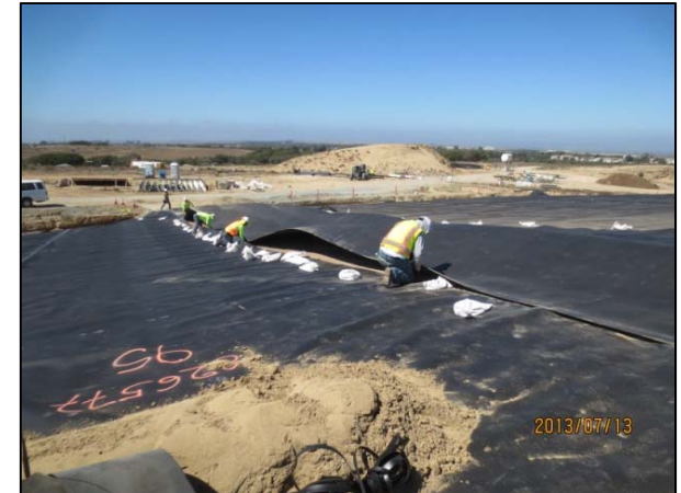
Joining geomembrane seams
