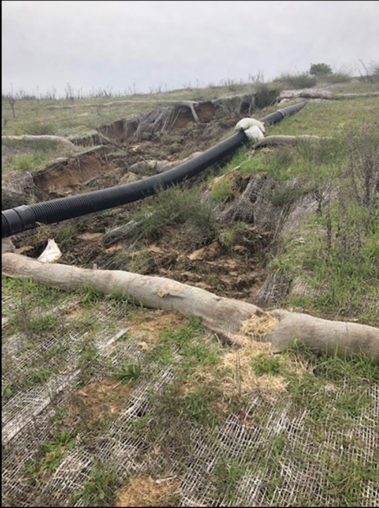
Area F vegetative cover erosion damage
