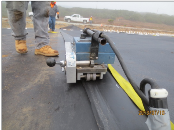
Welding geomembrane seams
