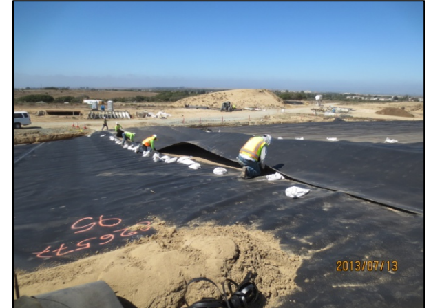
Joining geomembrane seams
