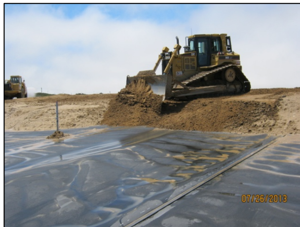
Placing vegetative cover soil
