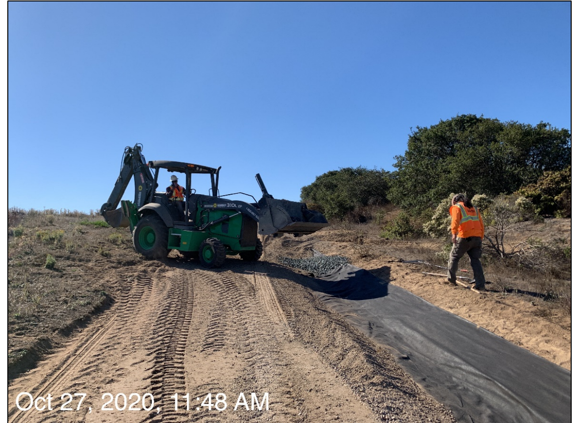
Perimeter Road Erosion Repairs
