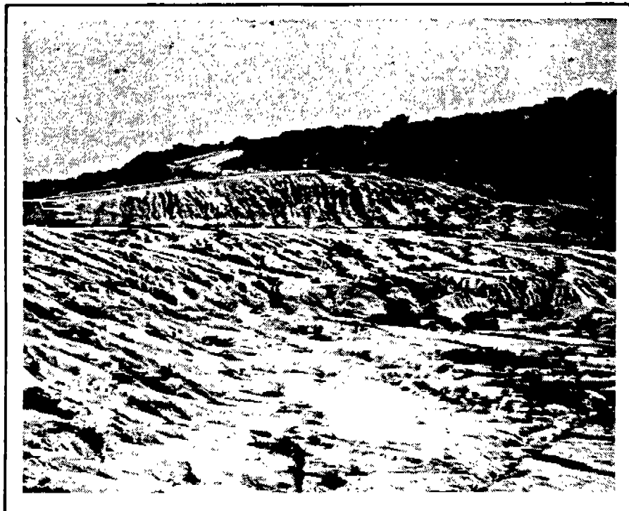
Erosion on cutbank and downslope of a roadway, Aromas formation on Fort Ord.
