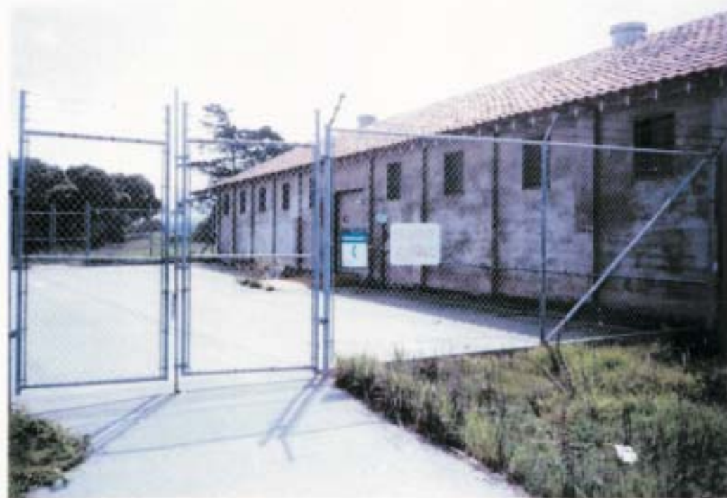
RCRA Unit FTO-009, DRMO PCB Storage (Building T-111)
