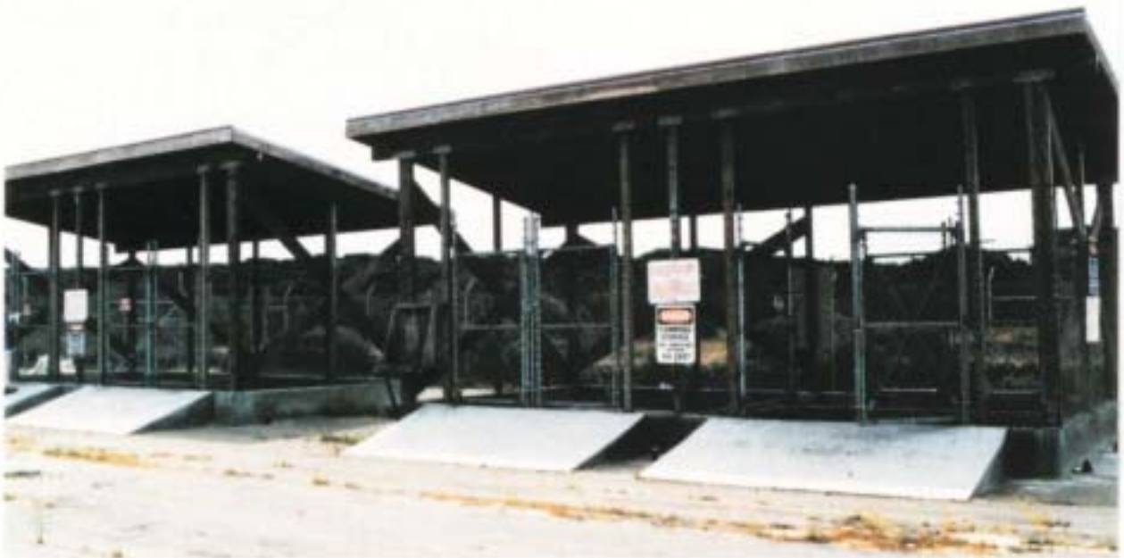
Site 20, FTO-066, Temporary Container Storage Units in Former Troop Training Area
