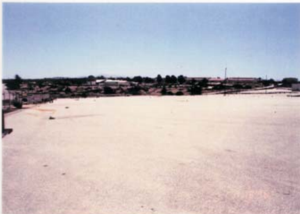
Site 17, FTO-065, RI/FS Site 17 Disposal Area, from northwest corner
