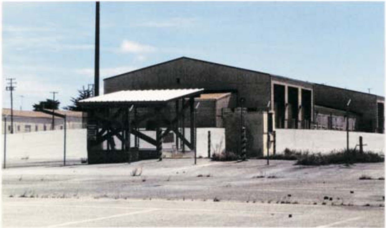
Site 18, FTO-041, 590th SS Company Motor Pool
