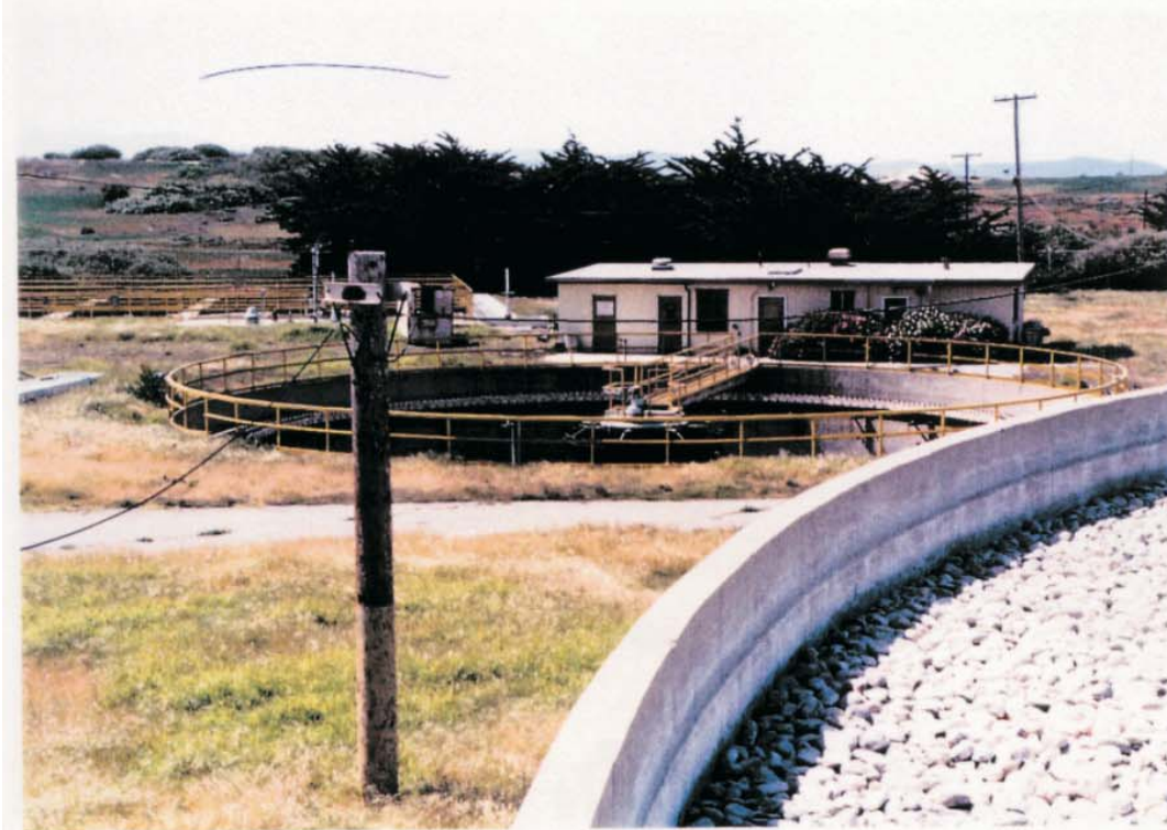
Site 2, FTO-012, Main Garrison Sewage Treatment Plant
