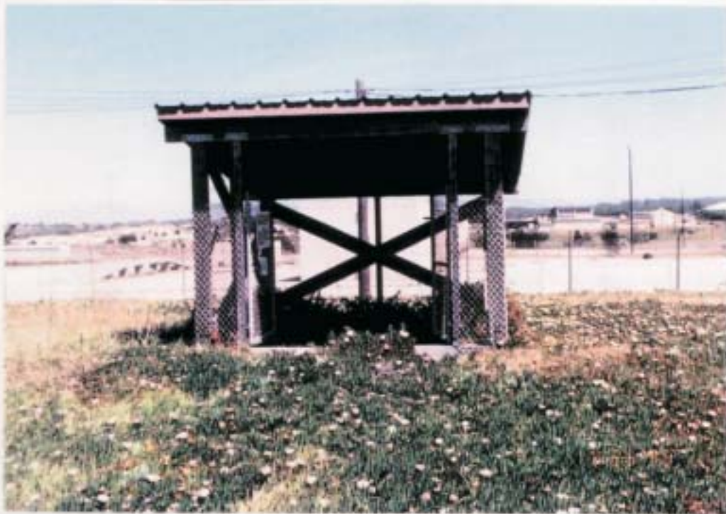
Site 17, FTO-064, Temporary Container Storage Unit Between Buildings 1458 and 1468
