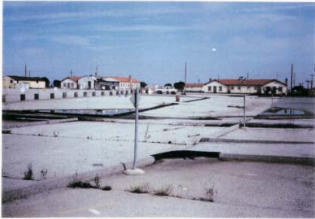
RCRA Unit FTO-008, DRMO Hazardous Waste Storage Area
