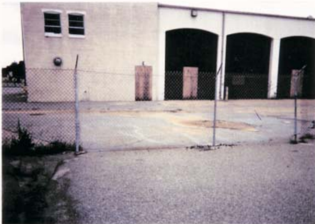
Site 18, FTO-044, 121st Aviation Battalion, Company E Motor Pool, Former Temporary Container Storage Unit
