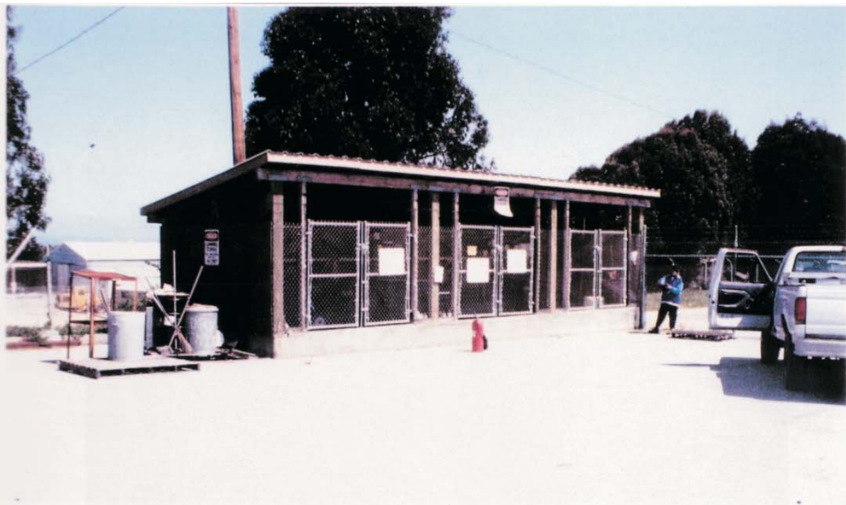
Site 14, FTO-004, 707th Maintenance Battalion, A, B, and C Company Motor Pools
