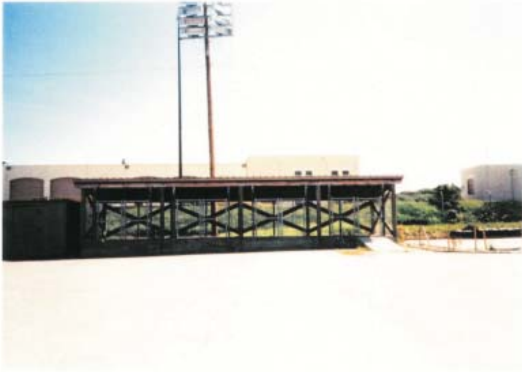
Site 22, FTO-025, 14th Engineer Battalion Motor Pool, looking east
