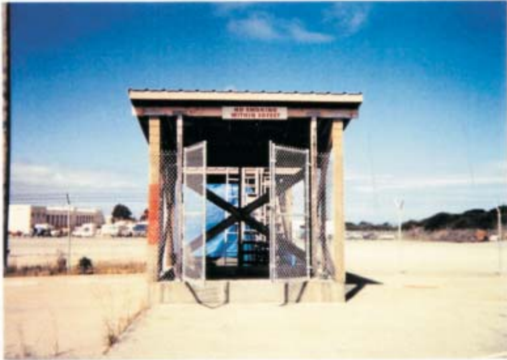
Site 21, FTO-032, 7th Aviation Battalion, C & D Company Motor Pool, looking west
