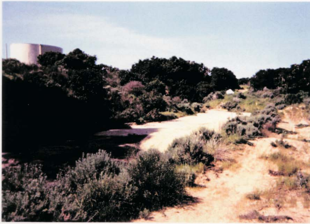
Site 32, FTO-011, East Garrison Sewage Treatment Plant
