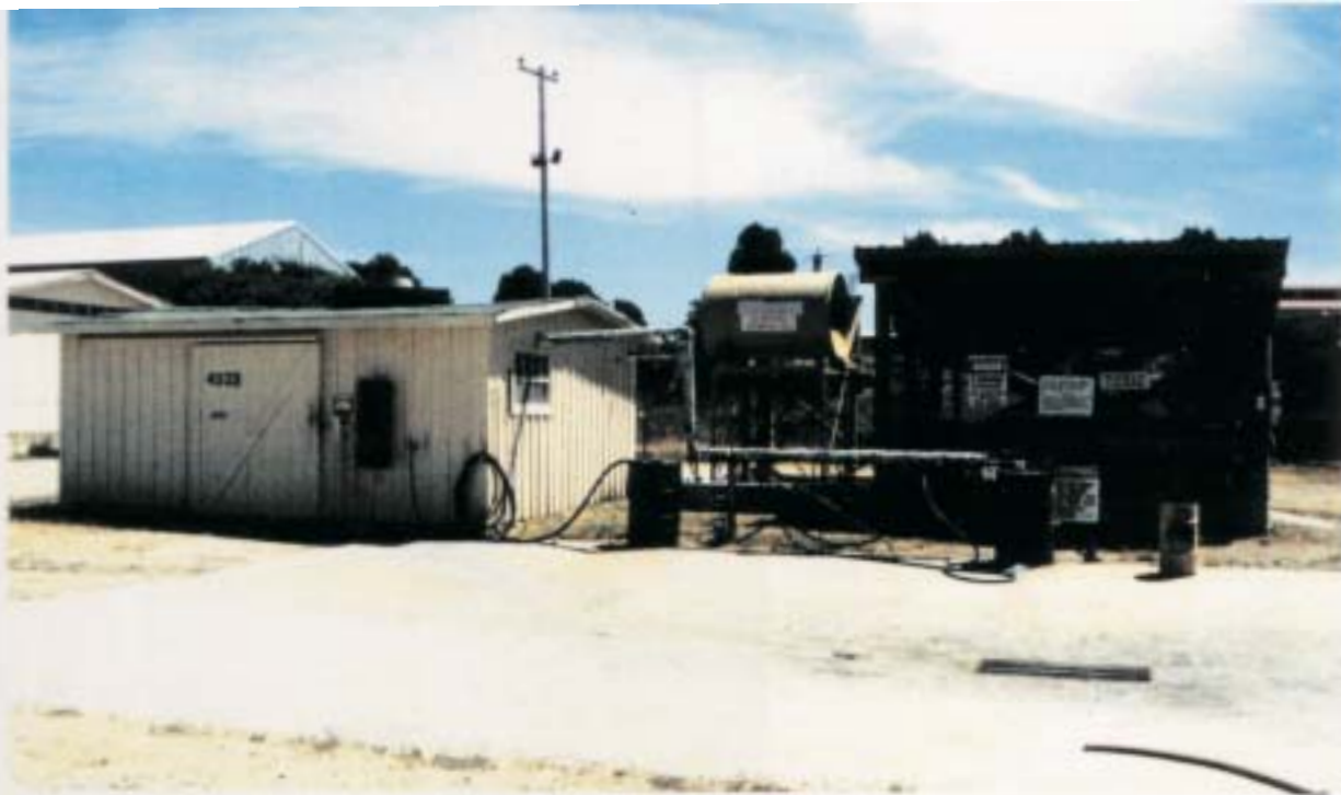
Site 16, FTO-036, DOL Heavy Equipment Maintenance Yard
