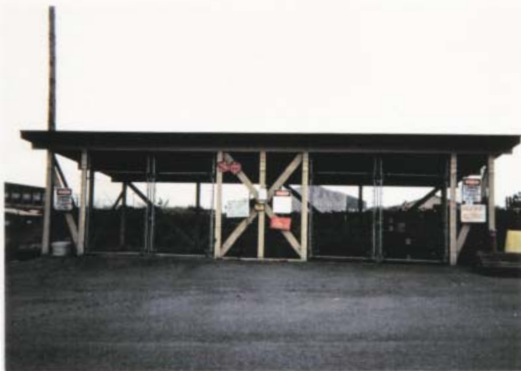
Site 15, FTO-015, Hazardous Waste and Equipment Storage Area
