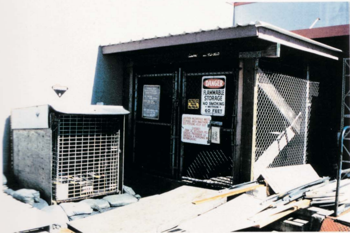
Site 11, FTO-010, AAFES Service Station, battery and waste storage cages
