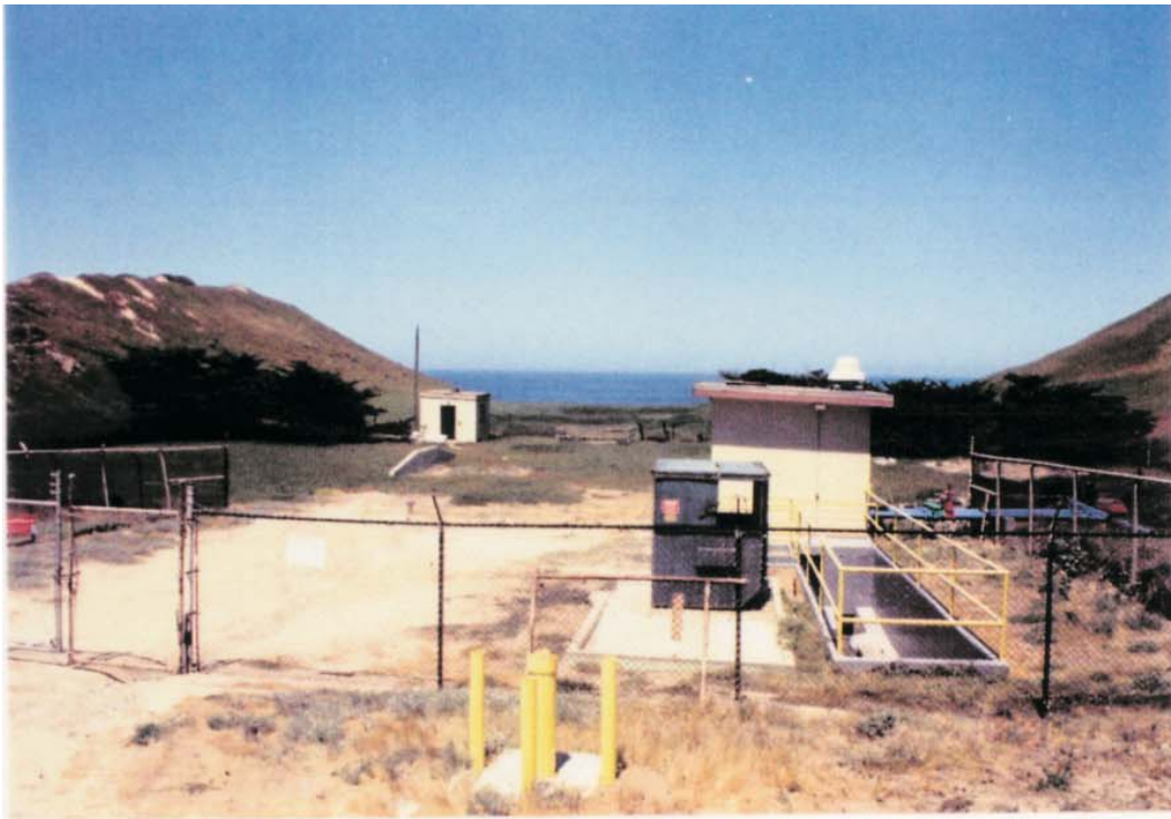
Site 1, FTO-059, Ord Village Sewage Treatment Plant
