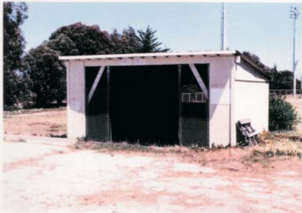
Site 17, FTO-063, Temporary Container Storage Unit East of Aces Carpentry
