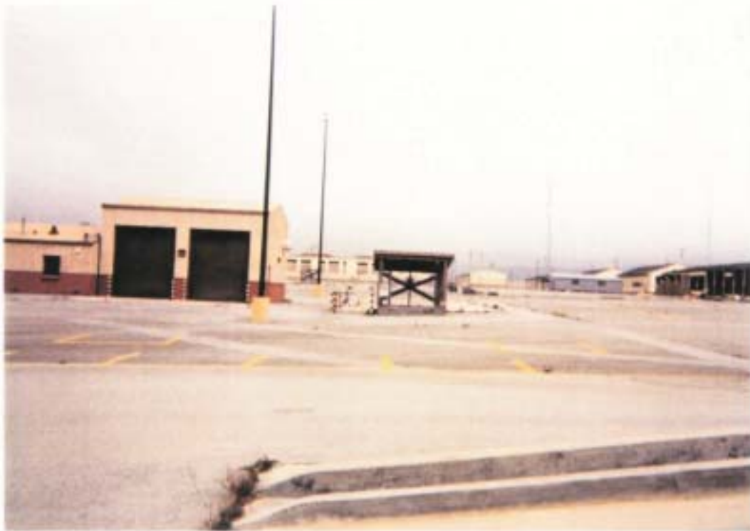
Site 18, FTO-057, 751st MP Company Motor Pool, looking east
