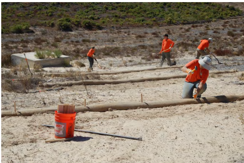
Figure 20. HA 28 wattle installation.
