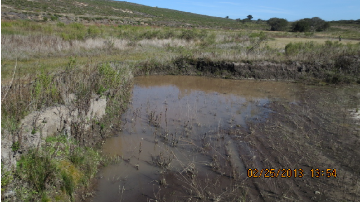
Photo 7. Remediation excavation depression Pool 30B on 25 February 2013. Water present.
