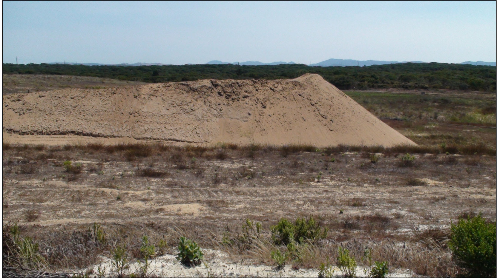
Stockpile of trench spoils from MCWD recycled water project.
