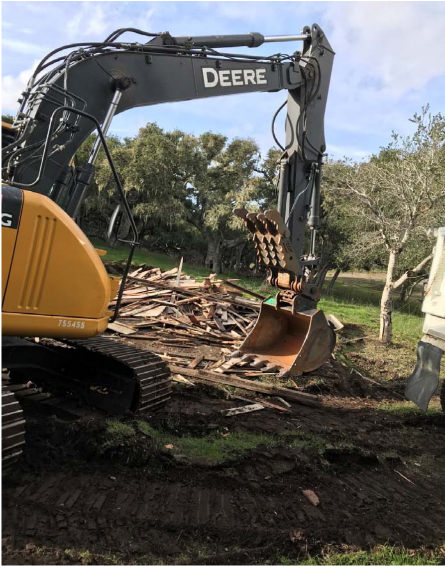
A) Demolition workers use an excavator BLM Area B, B3 West to break up and load out a latrine building.
