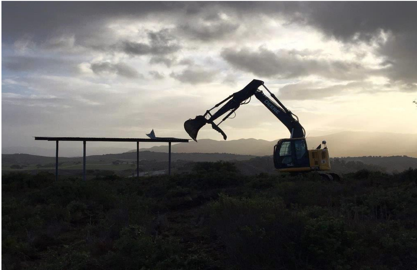
A) Excavator operator preparing to lower the canopy in Unit 9.
