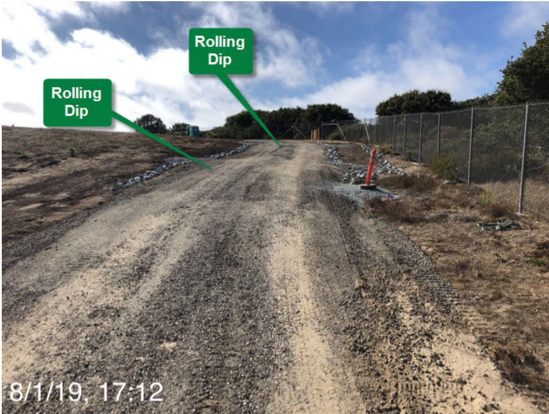
Perimeter Road Repair North Side Area F
