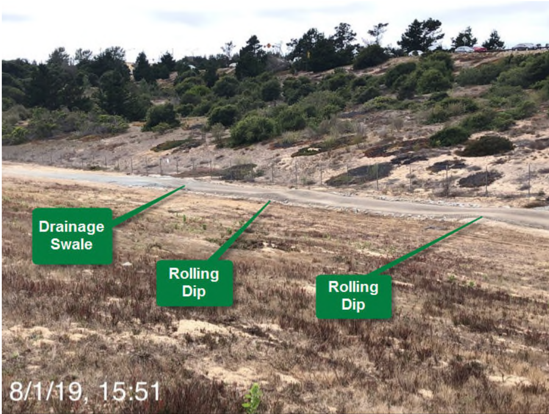
Perimeter Road Repair North Side Area B
