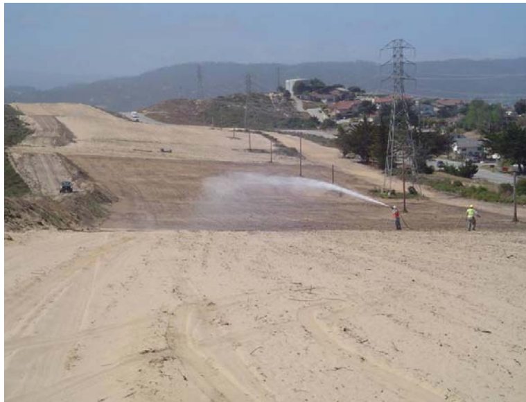
Photograph 3-24 – Soil Stabilization Activities to Minimize Wind Erosion
