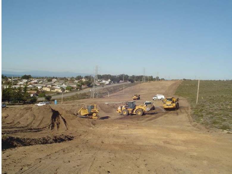
Photograph 3-8 – Clearing and grubbing operations within roadway alignment outside of SCAs
