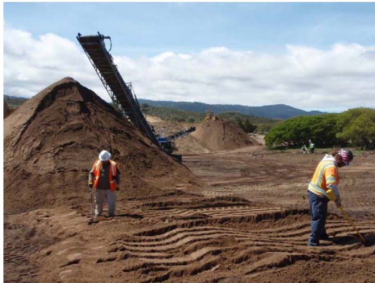
Photograph 3-18 – Inspection of sifted soil; Inspection was conducted twice daily for a portion of each stockpile of sifted soil generated
