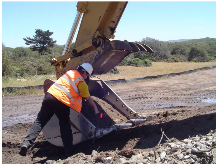
Photograph 4-1 – Placement of QC seeds into excavator bucket for feeding into sifting plant
