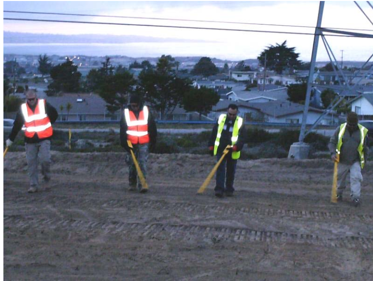
Photograph 3-10 – Instrument-aided visual inspection of roadway alignment during clearing and grubbing activities
