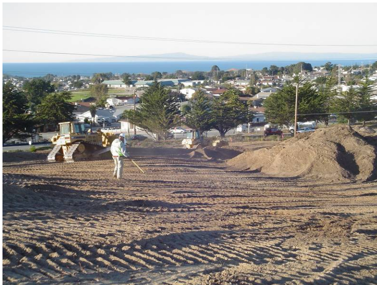
Photograph 3-9 – Instrument-aided visual inspection of the stockpiled soil during clearing and grubbing activities
