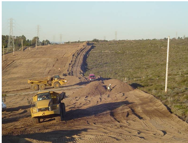
Photograph 3-11 – Instrument-aided visual inspection of cleared and grubbed roadway stockpile material
