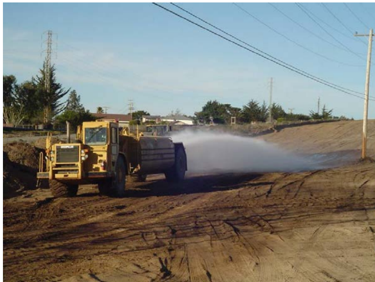
Photograph 3-23 – Water spraying activities to minimize fugitive dust
