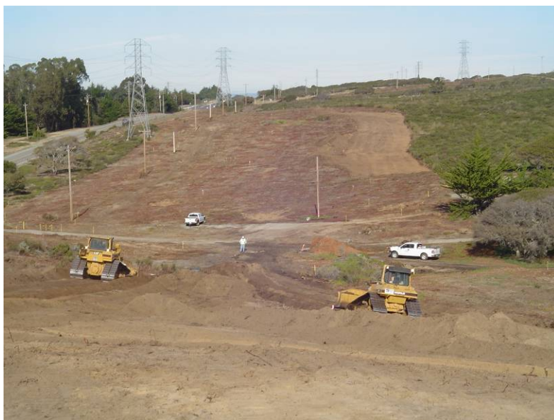
Photograph 3-7 – Clearing and grubbing operations within roadway alignment outside of SCAs.
