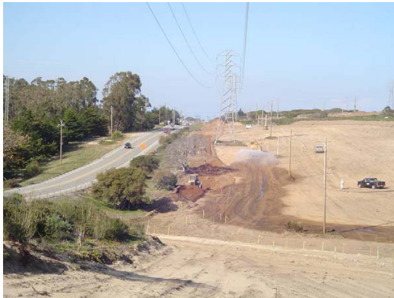
Photograph 3-13 – SCA polygon scraping and dust control activities
