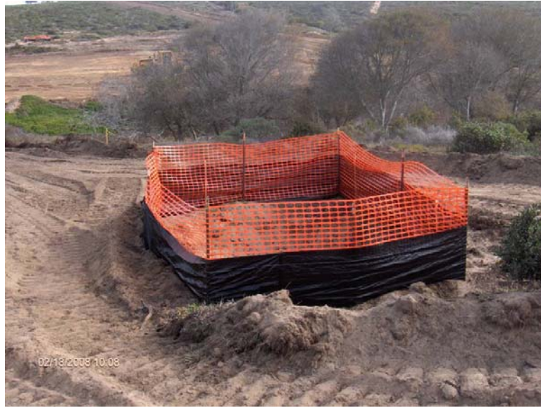
Photograph 3-21 – SCA excavation with silt fencing for protection of CTS
