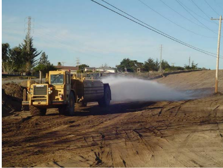
Photograph 3-23 – Water spraying activities to minimize fugitive dust
