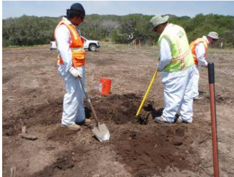
Photo 3-3 – Hand Excavation of Anomalies
