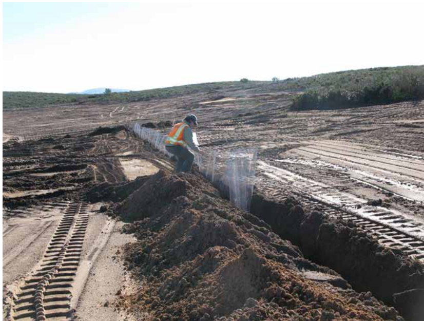
Photograph 8 – Interim Action Ranges MRA Range 47 Restoration Area. Below-ground fence installation to exclude burrowing animals. 7 January 2013
