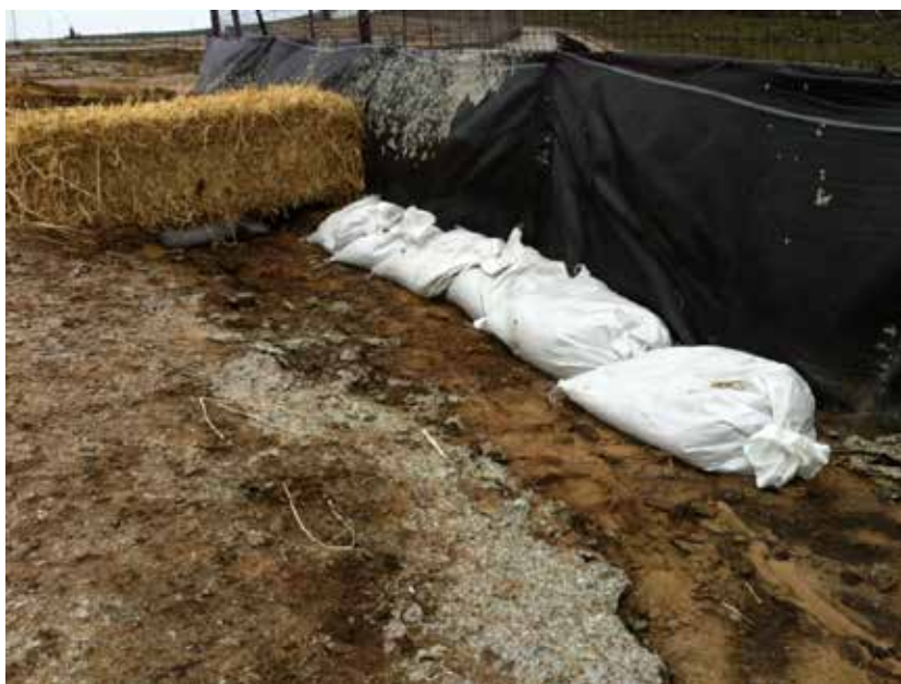
Photograph #4 – Silt fence – Section not properly buried, covered with sandbags
