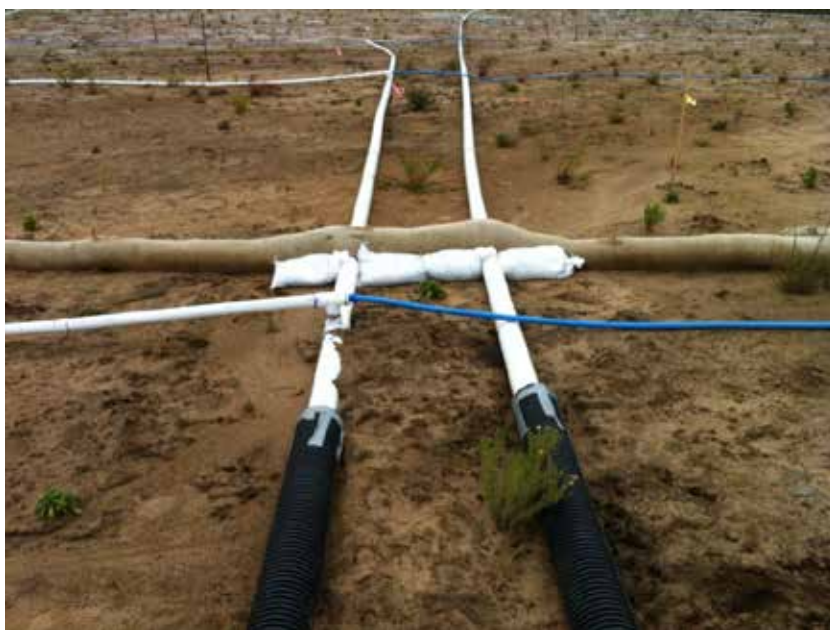
Photograph #2 - Straw wattles – gaps between irrigation lines, fixed with sandbags
