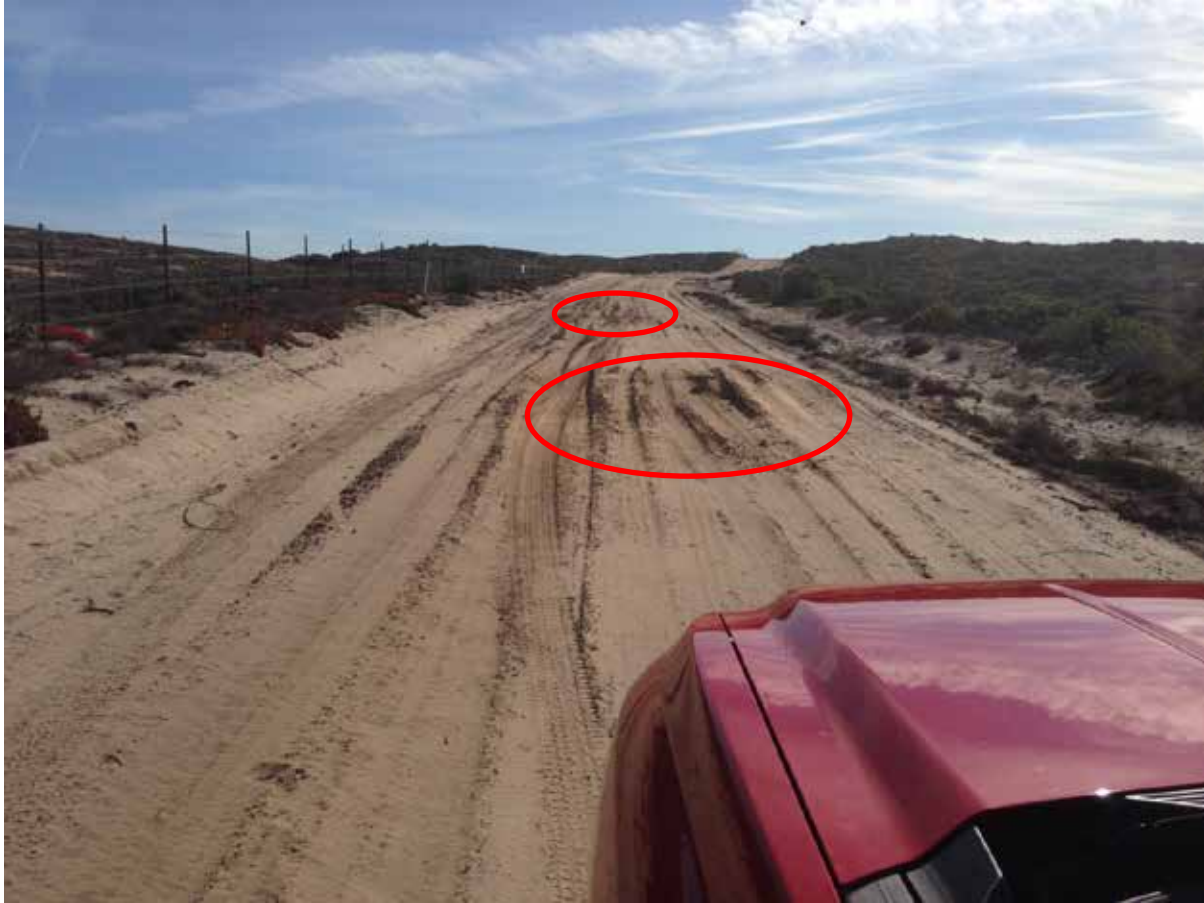
Photo 3. November 6, 2013 in Seaside MRA near Broadway West Gate. The road does not have sufficient crown to provide drainage to the sides. Generally recommended side-slope or crown slope is 4% to protect the road surface from erosion. Two circles show sunken areas with soft sand. During wet season these are at risk of erosion or of softening to the point of inhibiting vehicle passage.
