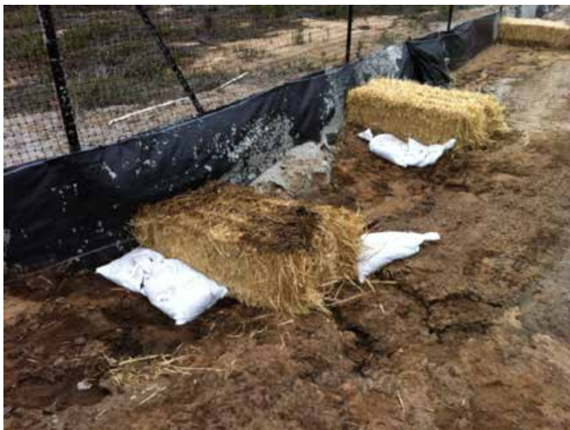
Photograph #6 – Straw Bales – Gaps under bales filled with sandbags
