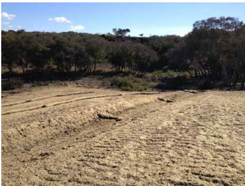
Photograph #6 Water bar and check dams in good repair
