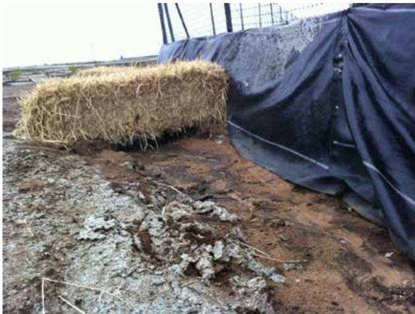
Photograph #3 – Silt fence – Section not properly buried
