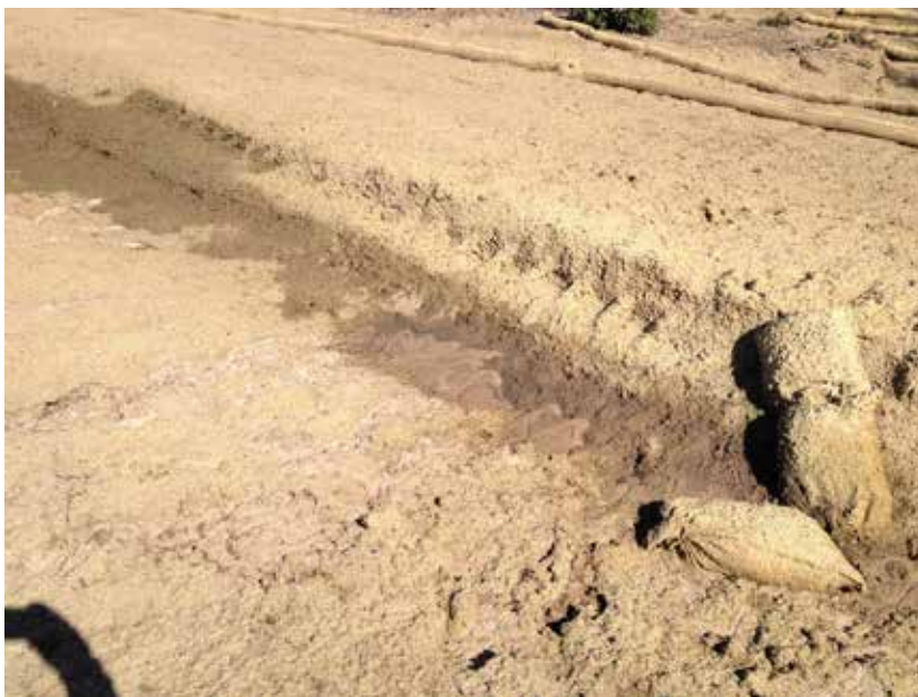
Photograph #4 – Check dams mid-gradient stopped sediment
