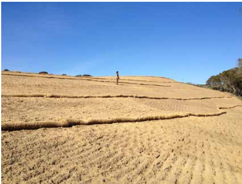
Photograph #5 Hydromulch and wattles in good repair
