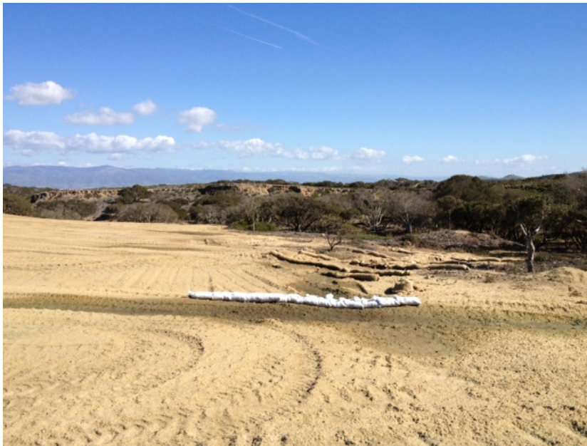
Photograph #1 – Sand bag repair for water bar
