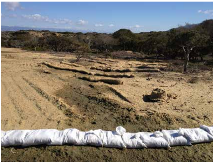
Photograph #3- Potential need for wattle replacement, but no new sediment observed
