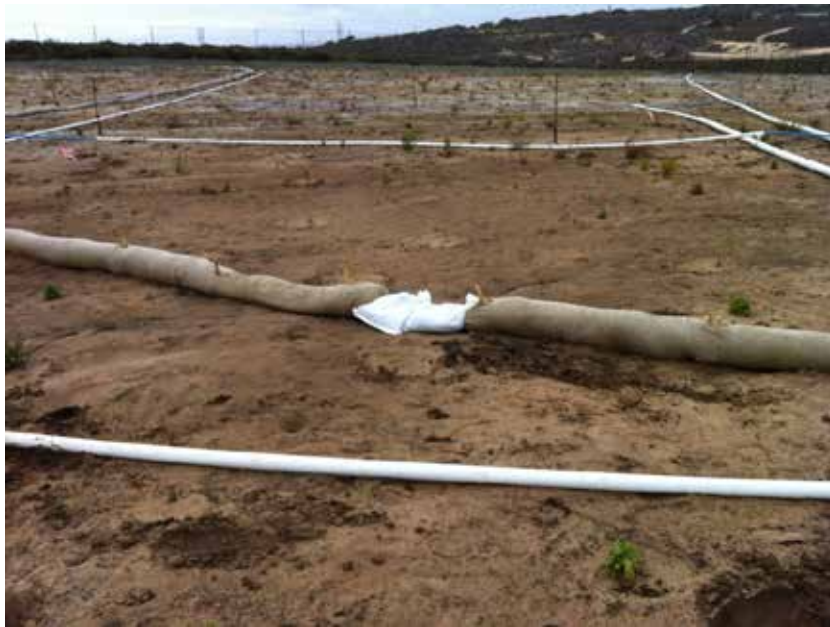
Photograph #1 – Straw wattles, - gap between run, fixed with sand bags
