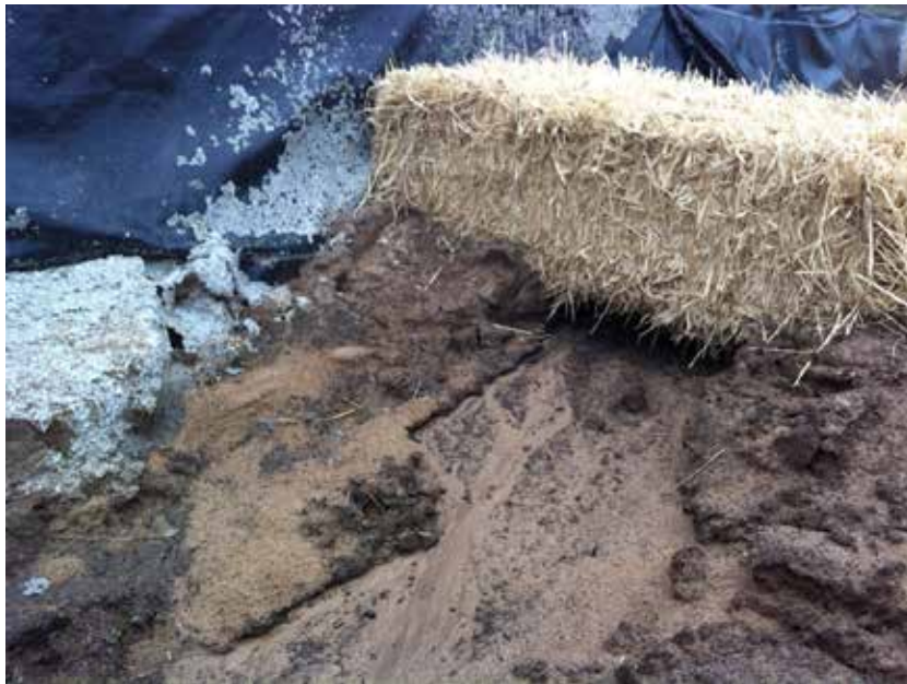
Photograph #5 – Straw Bales – Gaps under bales
