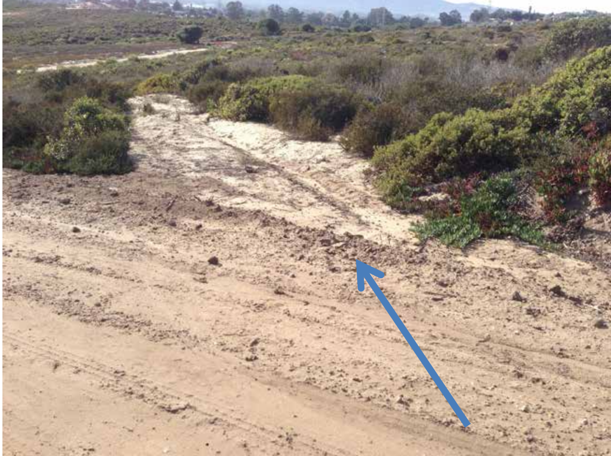
Photo 1. November 6, 2013 in southern Seaside MRA near Watkins Gate Rd. The road has developed a shoulder berm that prevents water from flowing in the direction of the arrow into the cross drain. The recommended erosion control practice is to remove the berm and create a rolling dip. Rolling dips should be cut deep enough to effectively divert water off the road, be backed up by a mound down slope, and be cut wide enough to easily pass traffic (50-100 feet). Department of Transportation specifications are discussed at http://ntl.bts.gov/lib/24000/24600/24650/Chapters/l_Ch7_Drainage_of_Low_Volume_Roads.pdf .
