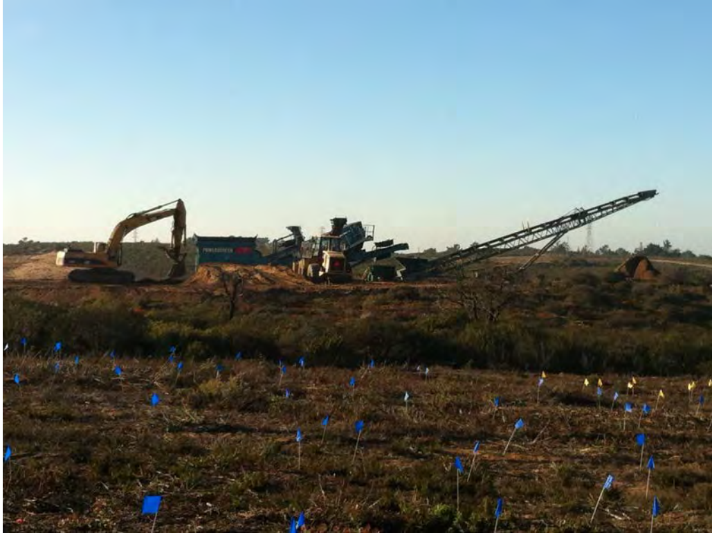
Picture 1: Sift operations at Range 47 IAR
