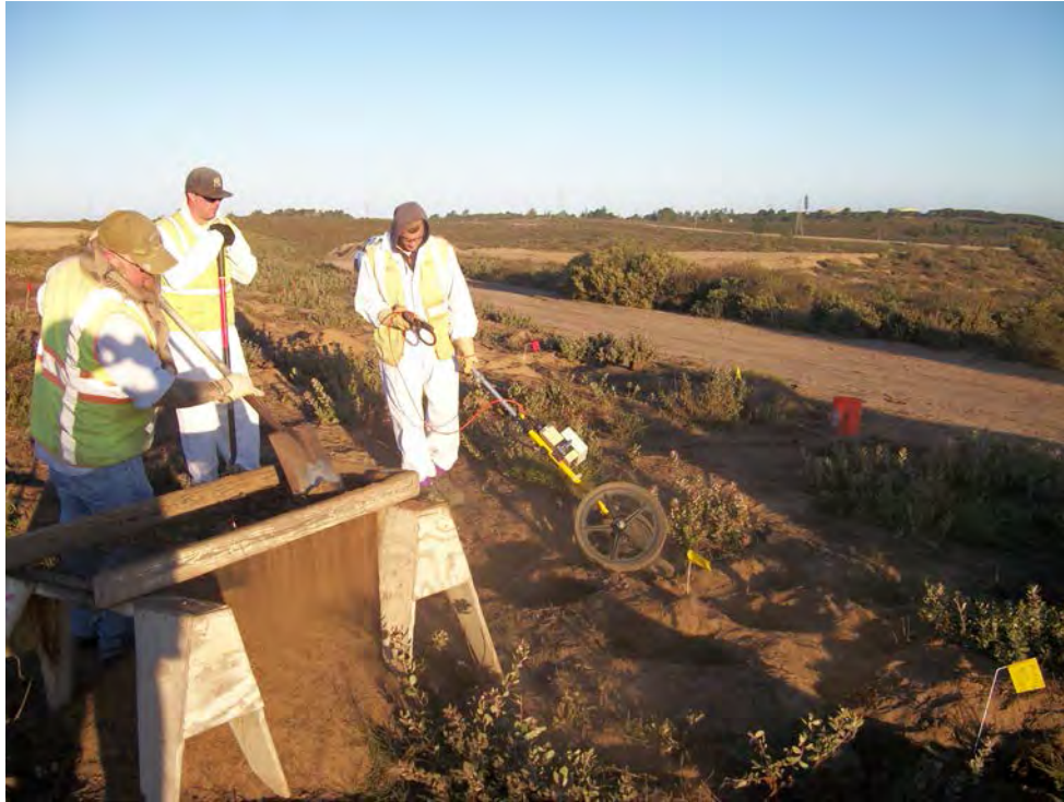
Picture 1: Sift table used in IAR 44 North SCAanomaly investigations
