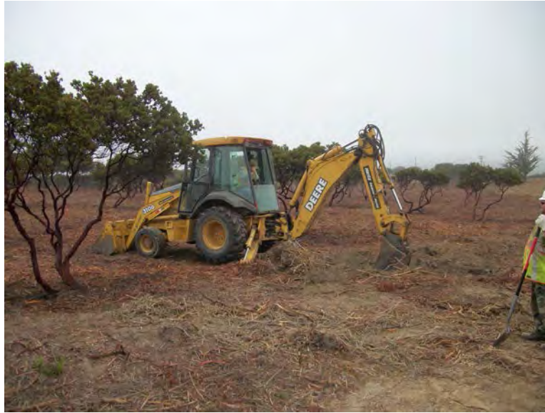
Pic 3: Backhoe operations in Future East Garrison parcel E11b.6.1.1
