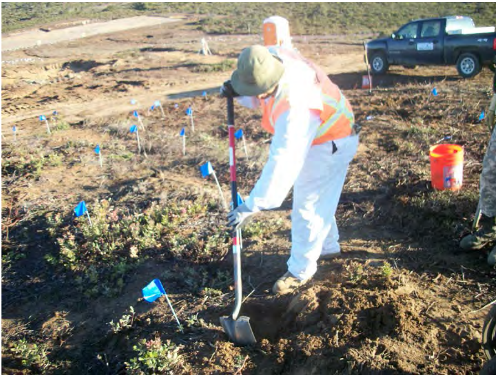
Picture 3: Anomaly excavation IAR R44 North SCA
