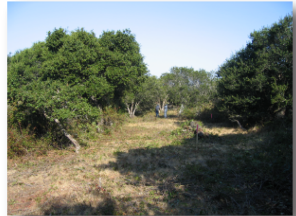
Photo 15. Well location IW-OU1-73-A after clearing looking south to north.
