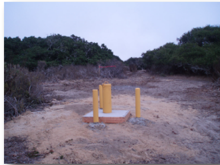
Photo 27. Finished well location MW-G (MW-OU1-82-A).
