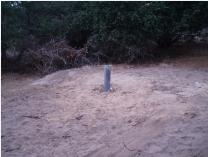
Photo 30. Well location IW-OU1-74-A after drilling was completed.
