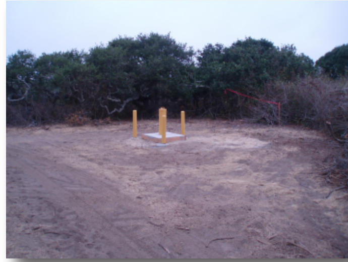
Photo 29. Finished well location MW-E (MW-OU1-84-A).
