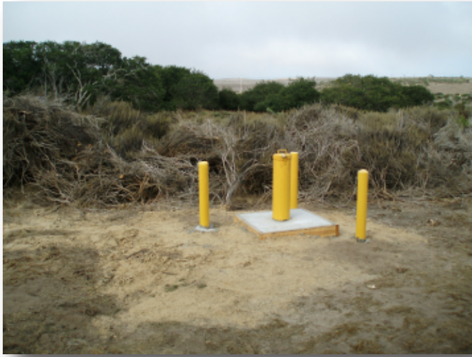
Photo 28. Finished well location MW-F (MW-OU1-83-A).
