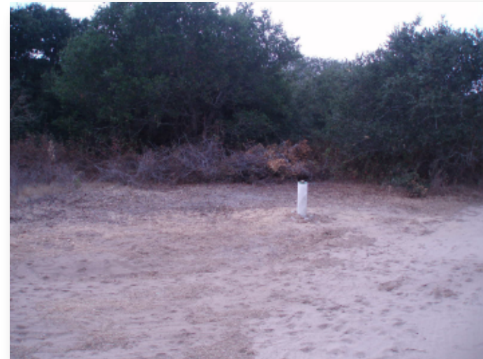
Photo 35. Well location MW-C (EW-OU1-87-A) after drilling was completed.
