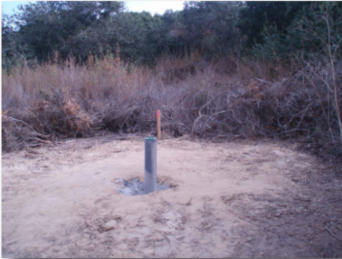
Photo 32. Well location MW-D (MW-OU1-85-A) after drilling was completed.
