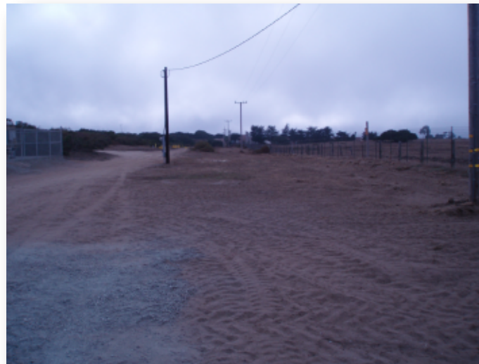
Photo 37. FONR staging area looking west after de-mobilization.
