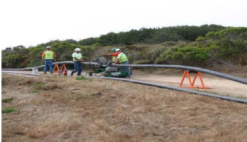
Photograph 1.2 – Laying out high density polyethylene pipe along the pipeline route.
