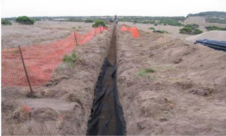
Photograph 1.3 – Excavation for injection trench.
