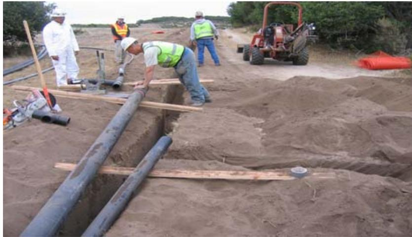
Photograph 1.1 – Trench excavation with ditch witch in background.
