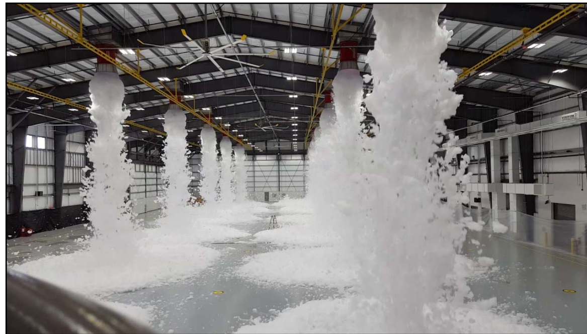
Example high expansion foam generator
