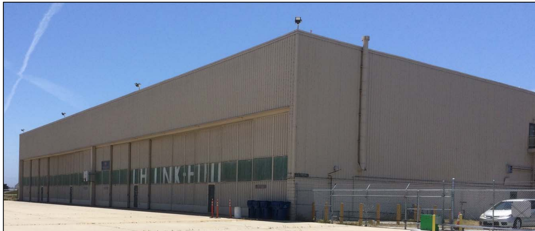
Building 527 north exterior view.
