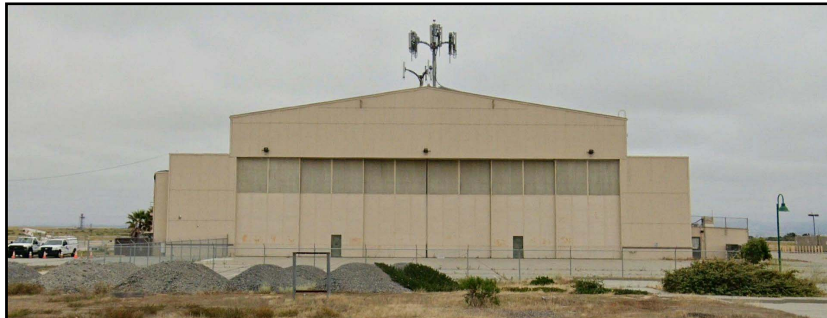
Building 524 south exterior view.
