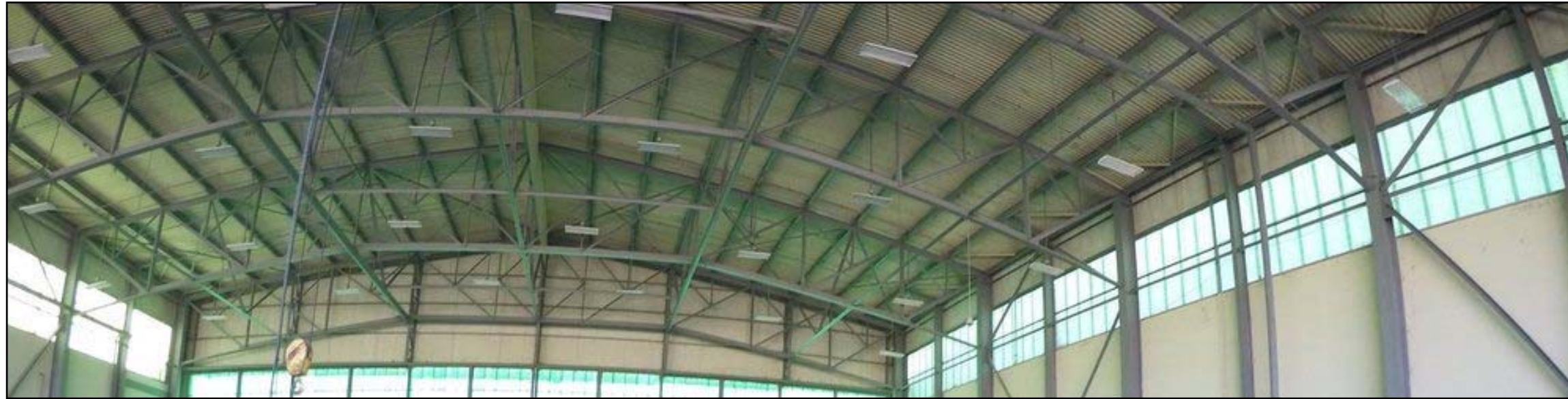
Building 533 south interior view.
