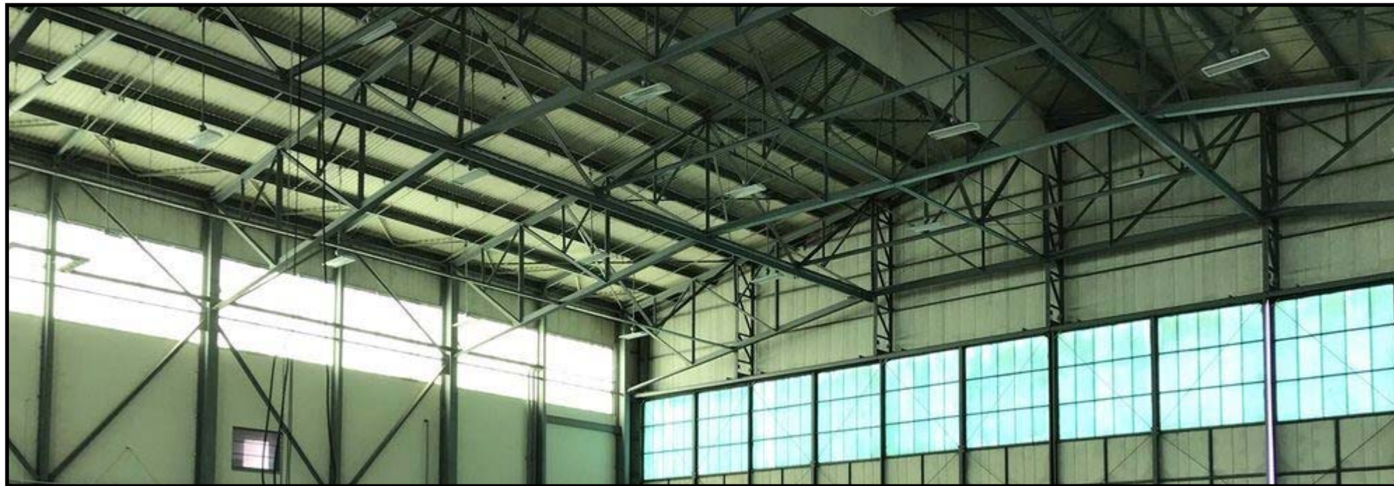
Building 533 north interior view.
