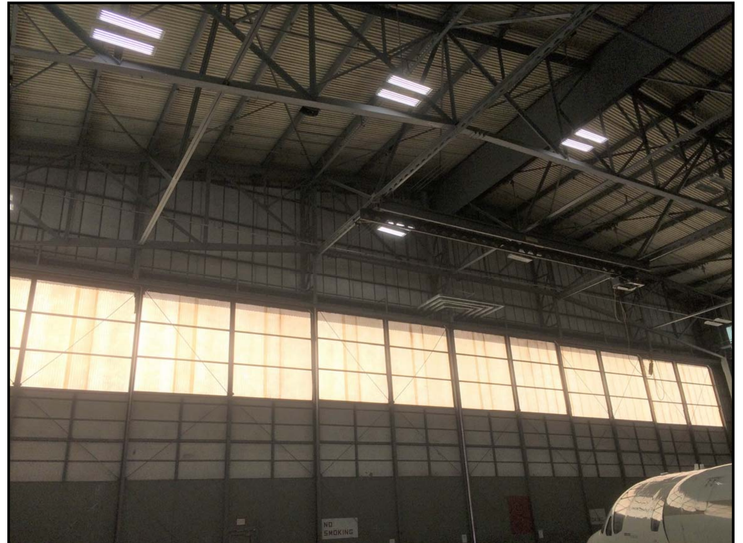
Building 524 south interior view.
