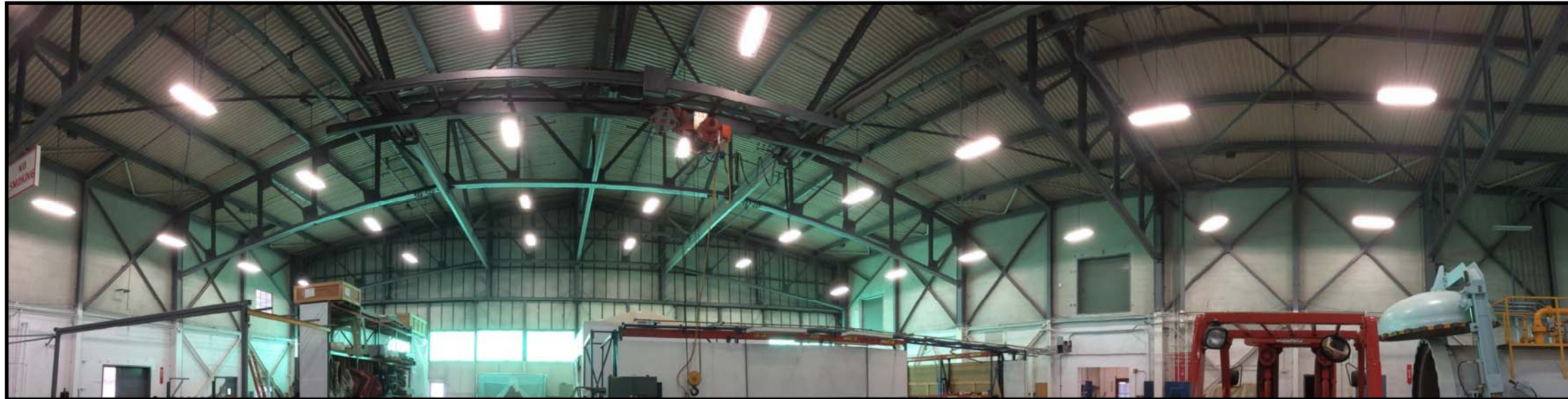
Building 510 southwest interior view.
