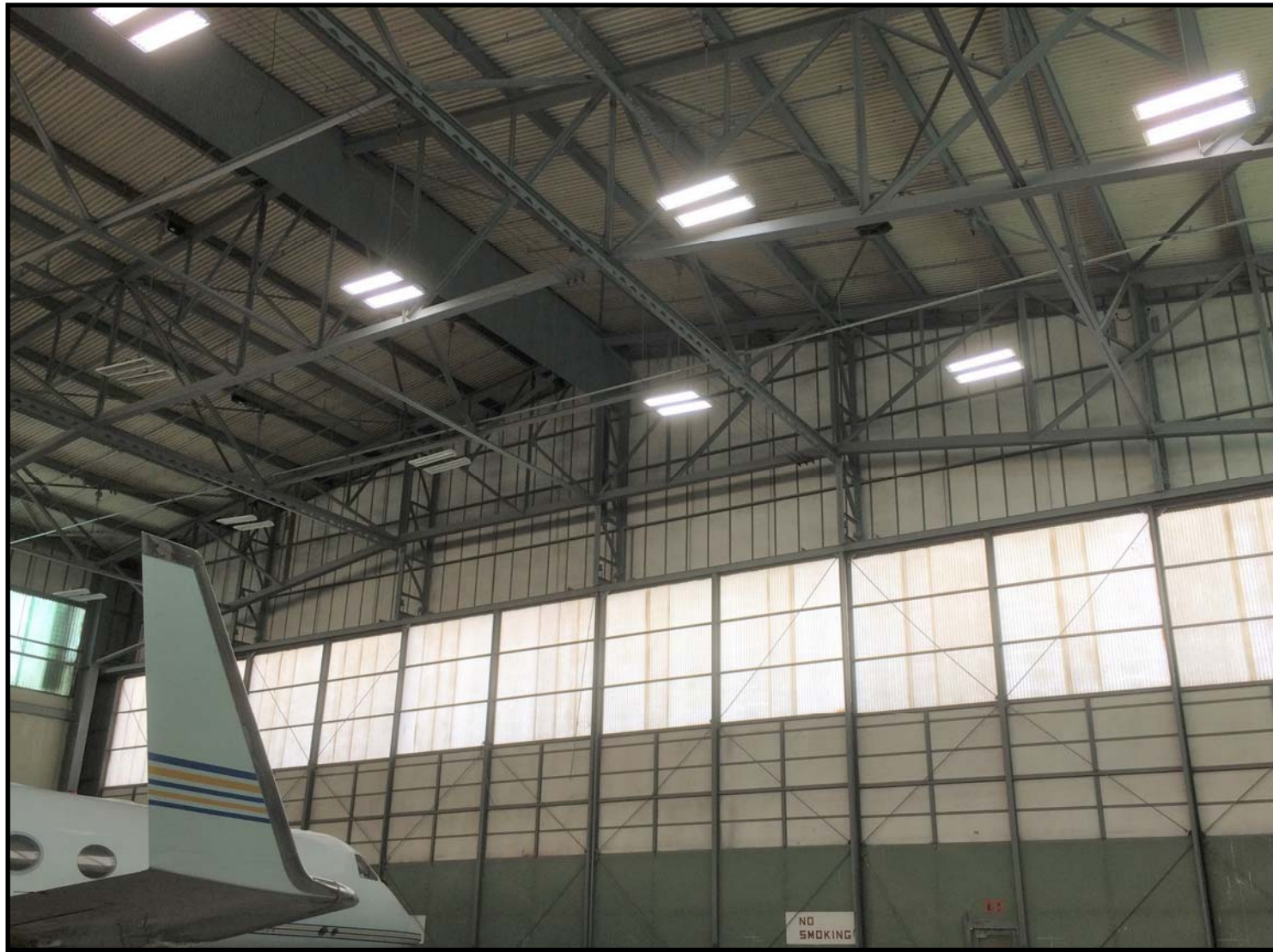
Building 524 north interior view.
