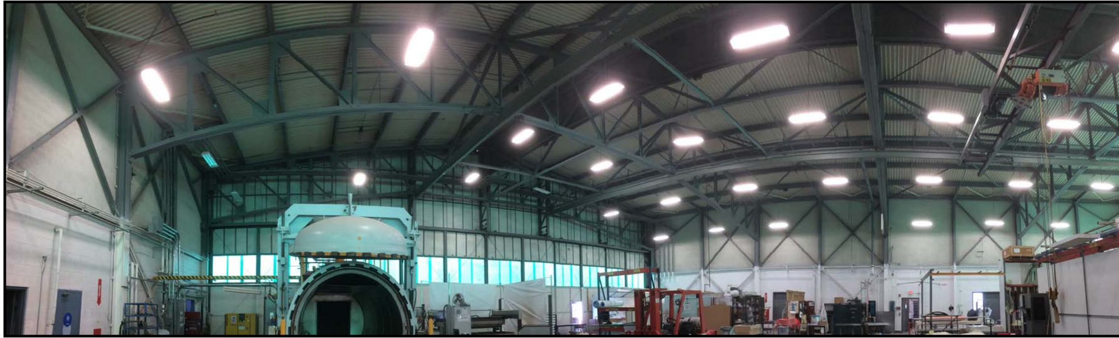
Building 510 northeast interior view.
