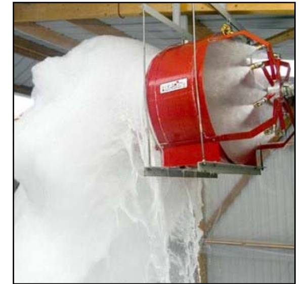
Example high expansion foam generator
