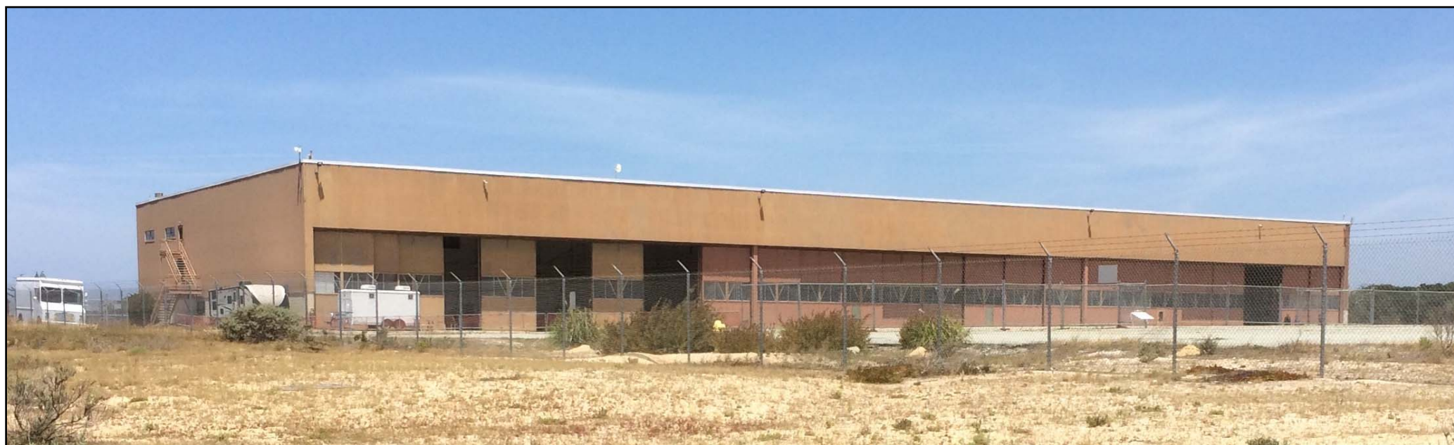
Building 507 north exterior view.
