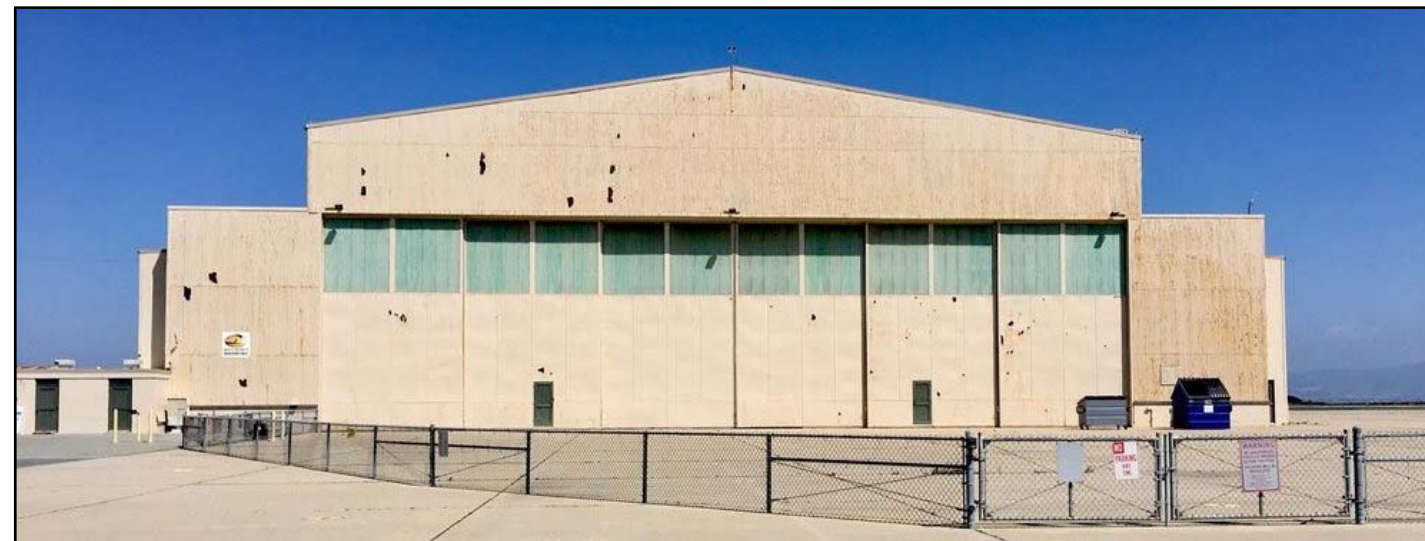
Building 533 north exterior view.
