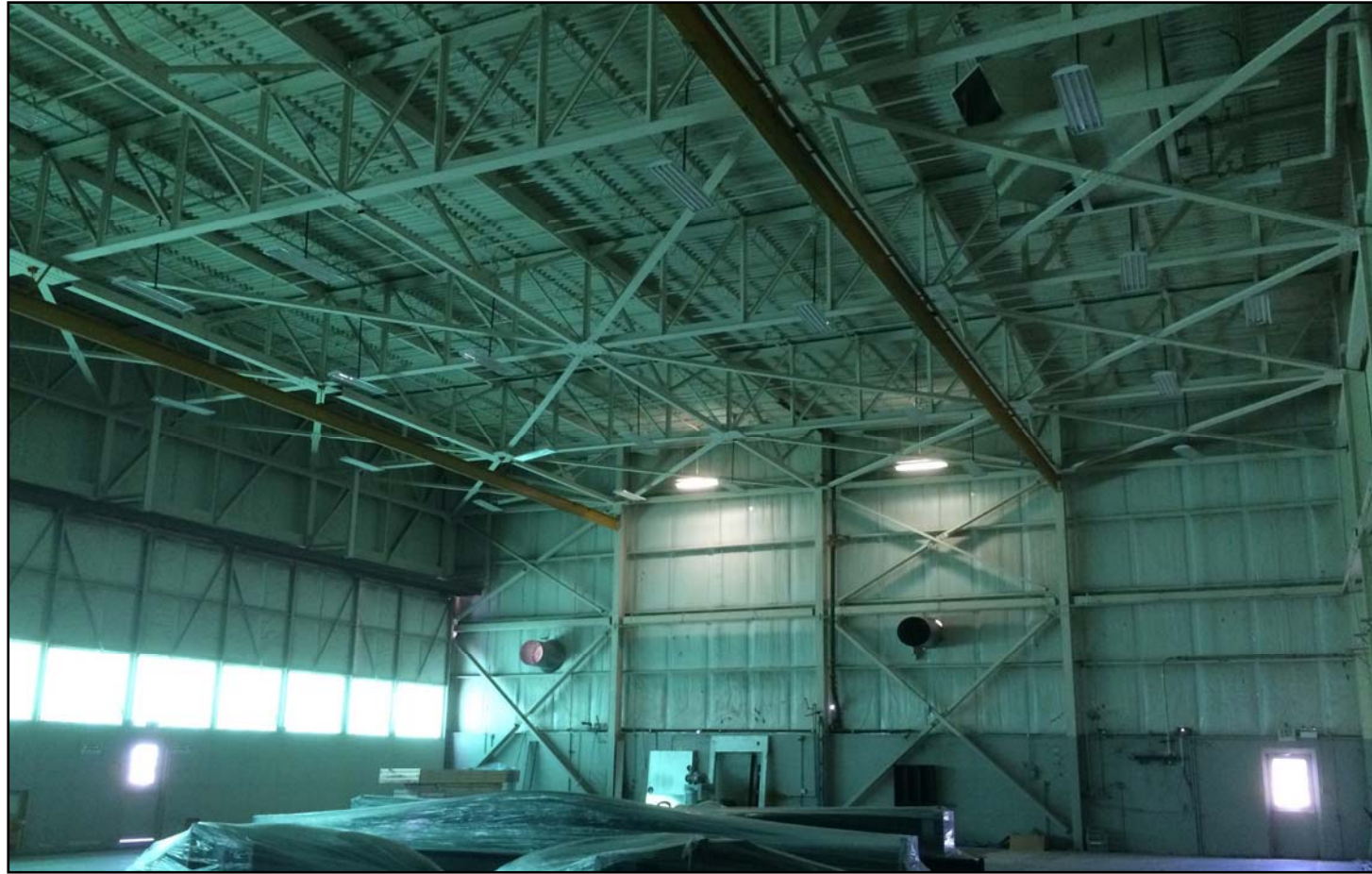
Building 527 east interior view.
