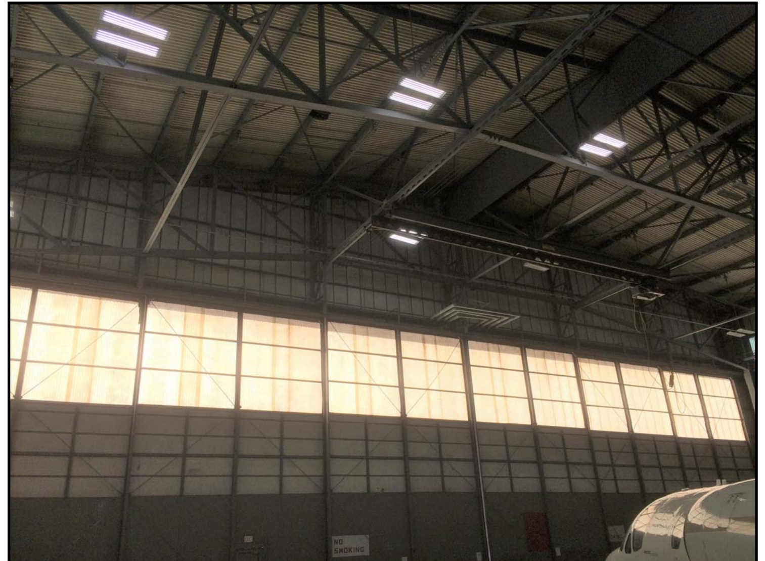
Building 524 south interior view.
