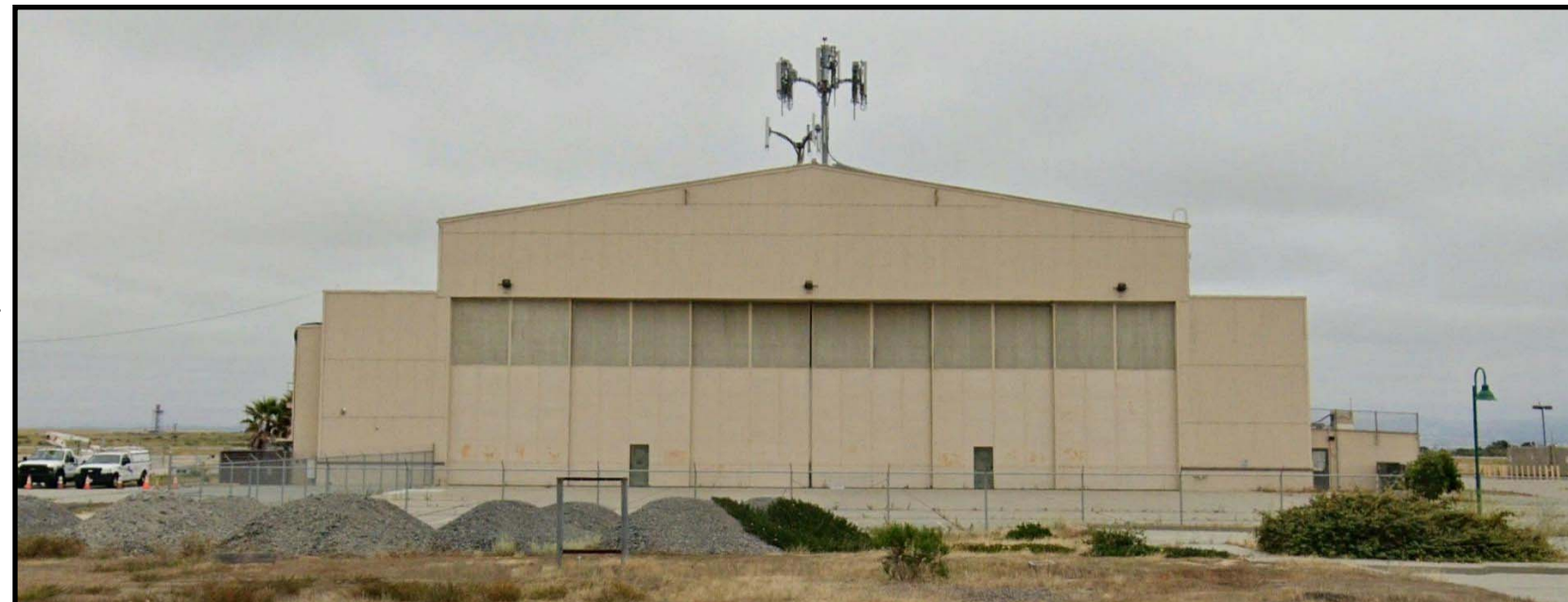
Building 524 south exterior view.
