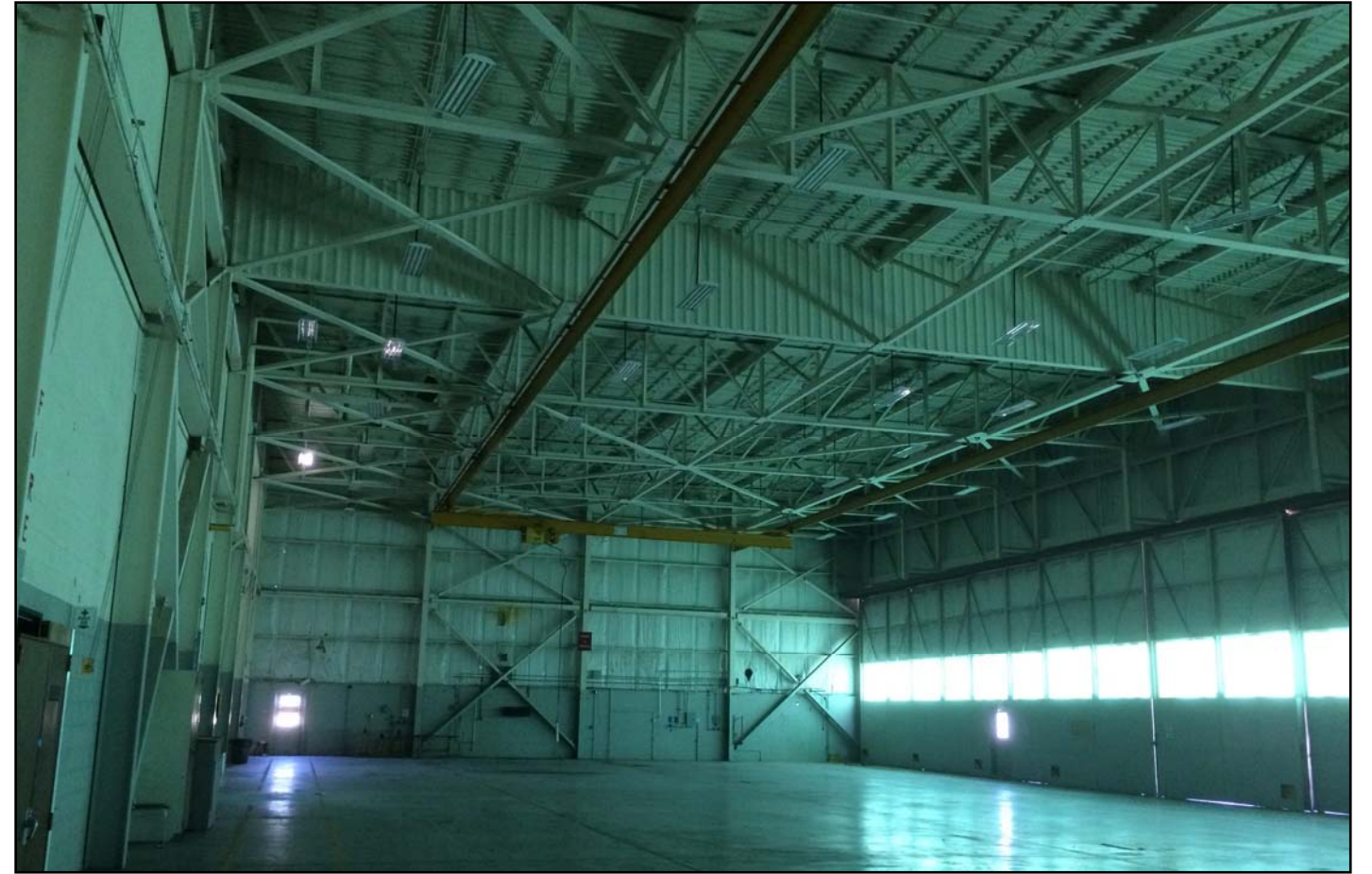
Building 527 west interior view.
