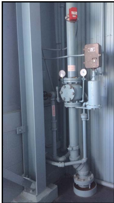
FAAF hangar support area wet system valve (typical)
