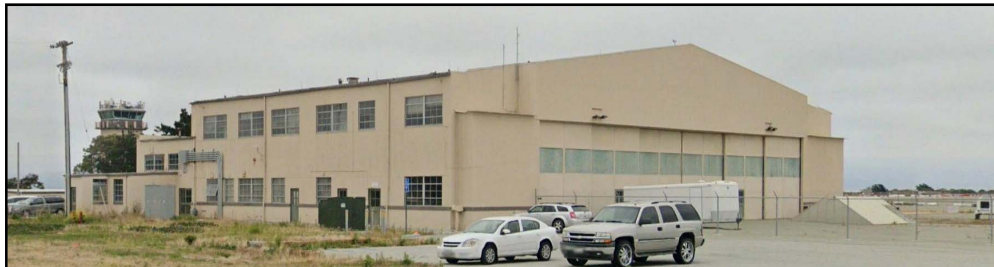
Building 510 west exterior view.
