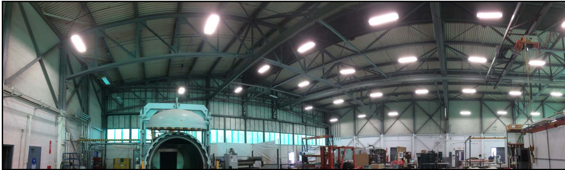
Building 510 northeast interior view.
