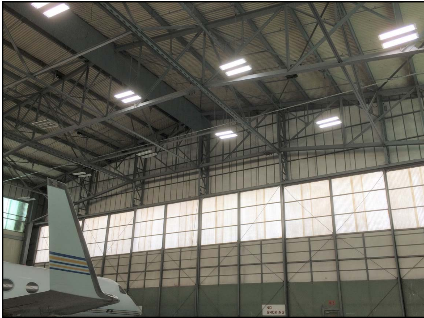
Building 524 north interior view.
