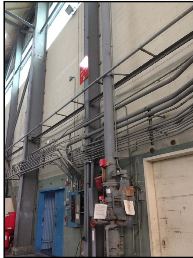
FAAF hangar water deluge valve system and riser pipe (typical)
