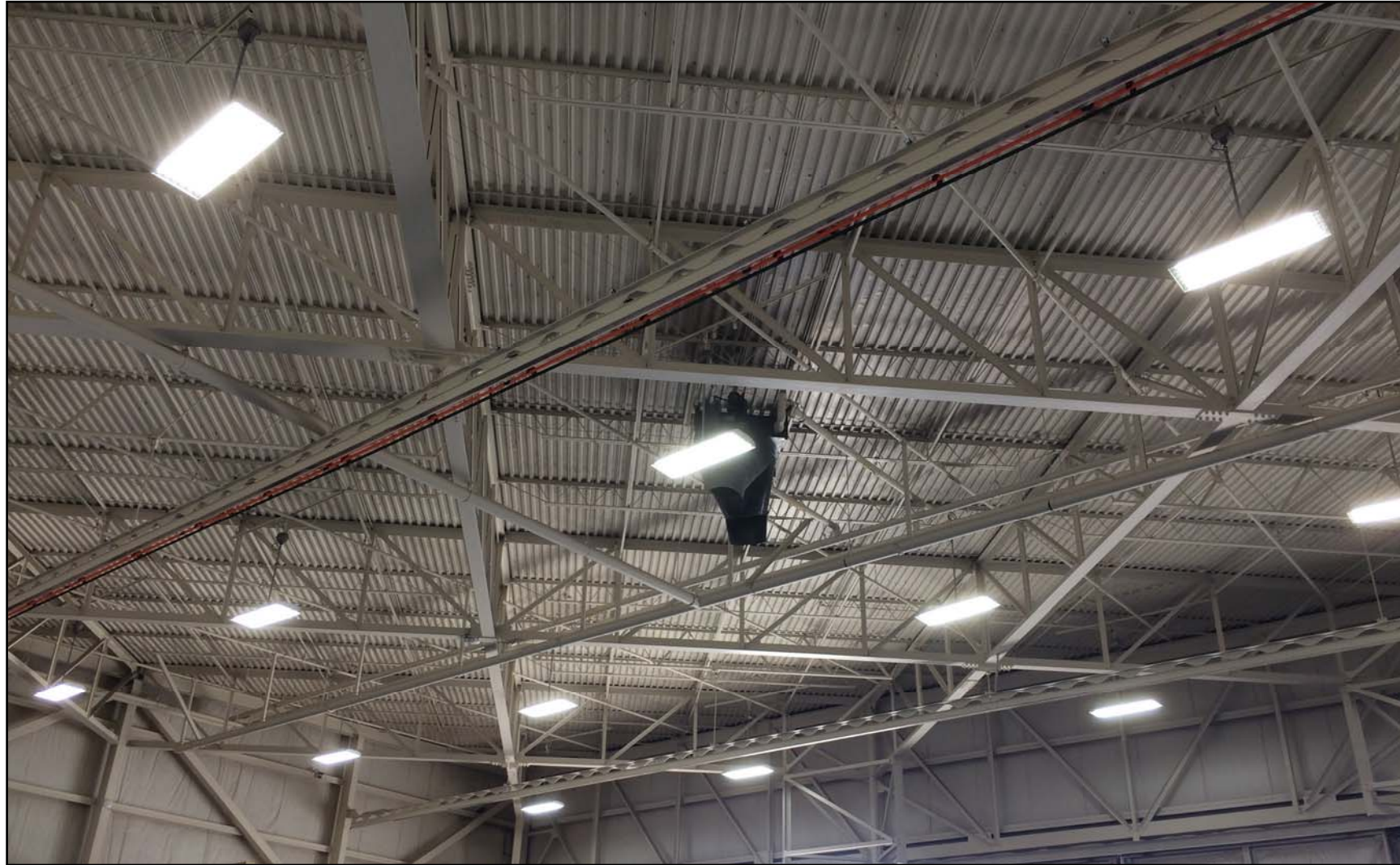
Building 507 suspected high expansion foam generator in hangar.
