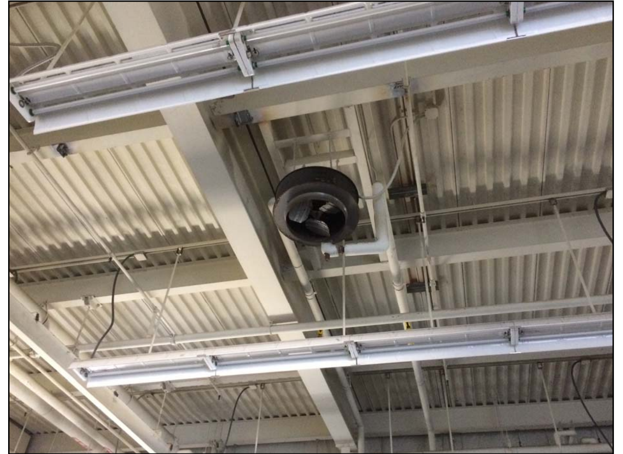
Building 507 suspected high expansion foam generator in storeroom/workshop.
