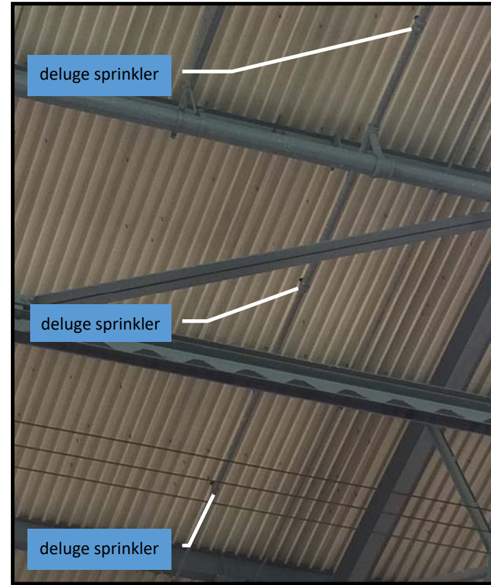
FAAF hangar water deluge sprinkler system (typical)
