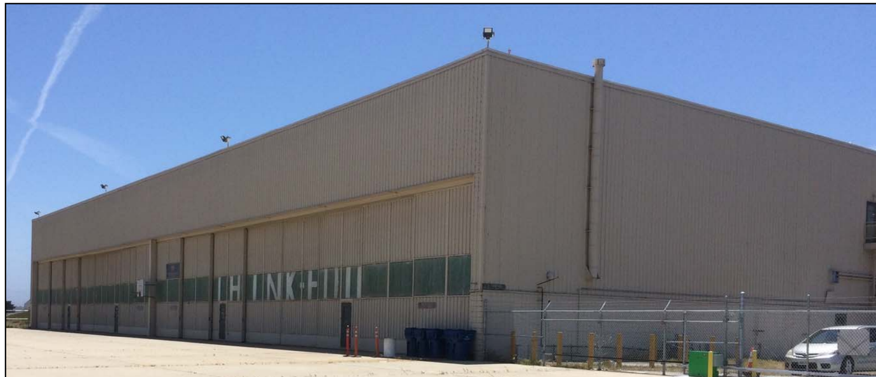
Building 527 north exterior view.
