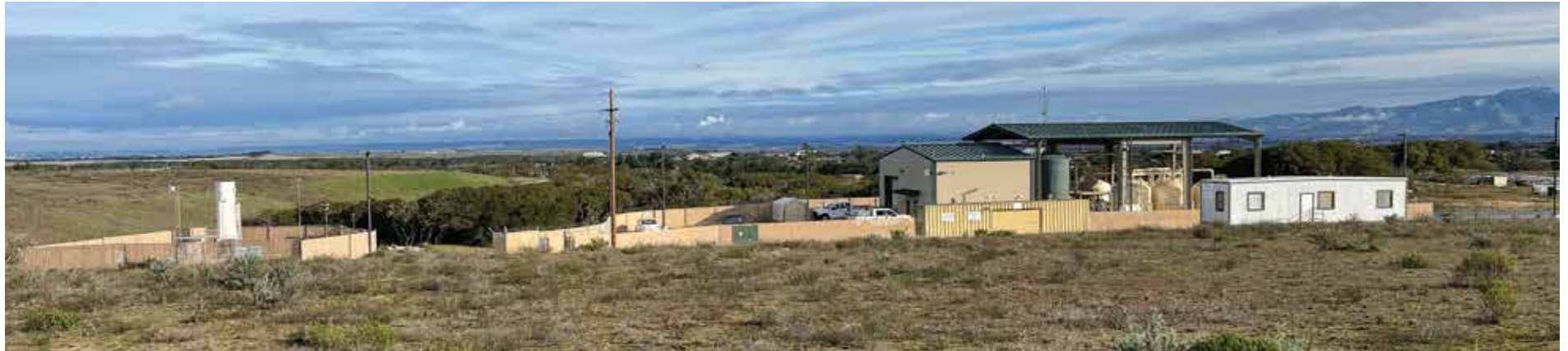
Operable Unit 2 Groundwater Treatment Plant
