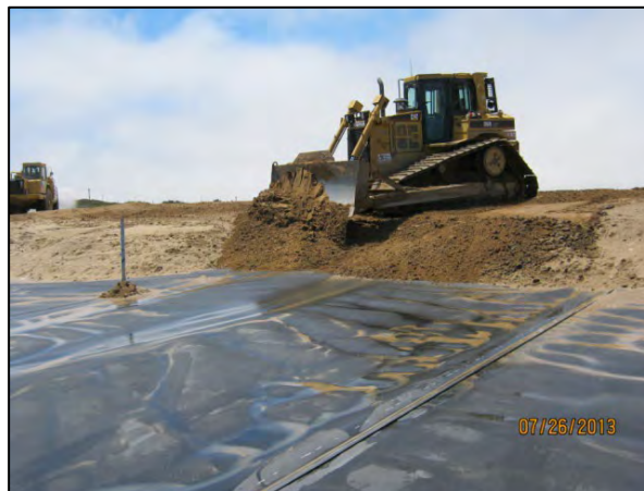
Placing vegetative cover soil
