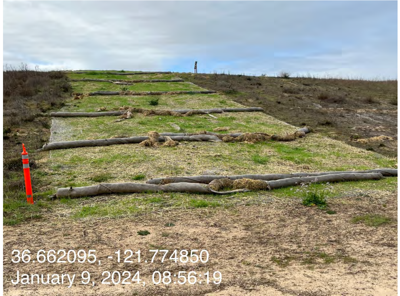
Area F vegetative cover erosion repairs
