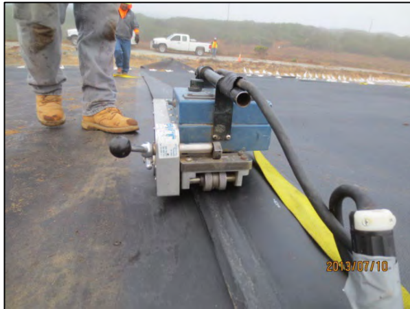
Welding geomembrane seams
