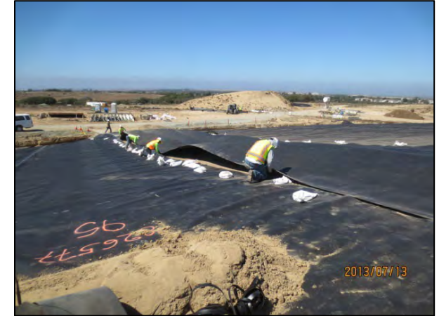
Joining geomembrane seams
