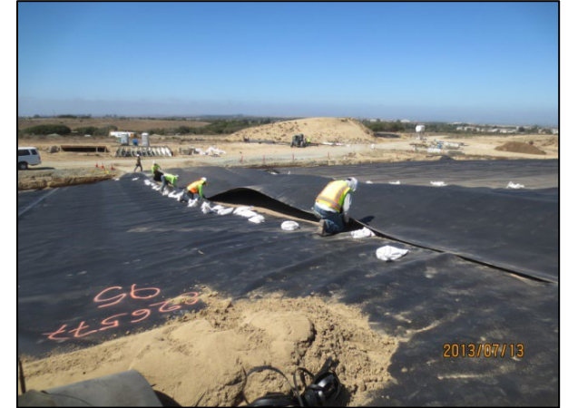
Joining geomembrane seams
