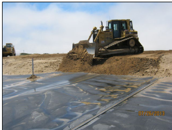
Placing vegetative cover soil
