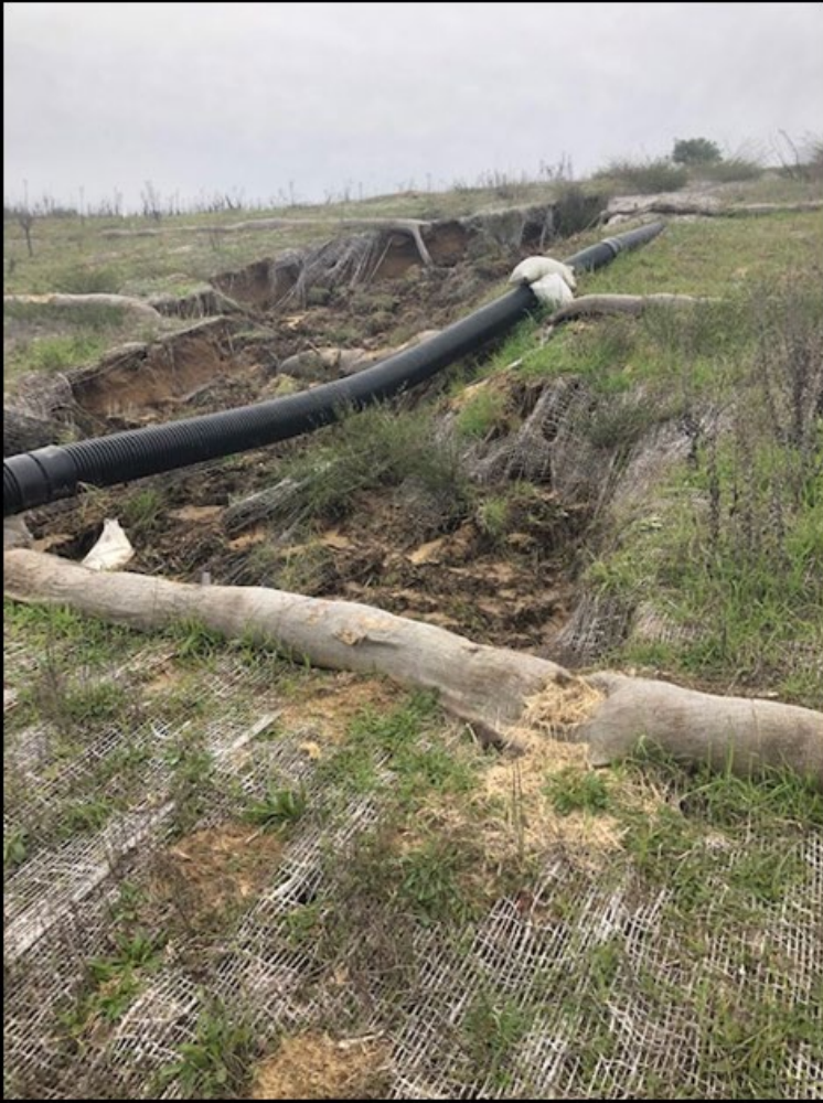
Area F vegetative cover erosion damage
