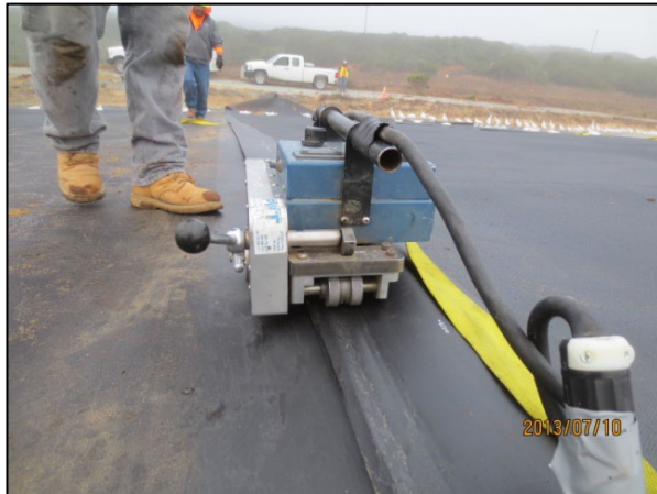
Welding geomembrane seams
