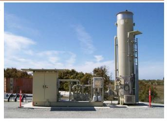
and potentially hazardous trace gases collected from under the cover of the landfill. The Army is operating the treatment system to maintain the methane concentrations in the soil at the landfill perimeter at acceptable levels and to remove chemicals that might otherwise migrate to groundwater.
