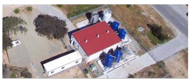
The OU2 Groundwater Cleanup System: A Closer Look Above is a photo of the OU2 treatment plant built in 1995. The blue tanks shown above are filled with activated carbon and are used as part of the OU2 treatment system to clean up contaminated groundwater. This plant will eventually be relocated to an area near the landfill.
