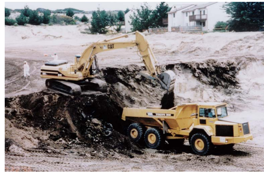
Excavation of wastes from Area A in 1996. The wastes were transported in trucks across Imjin Road and placed in the other areas of the landfill.
