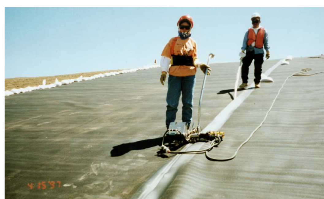
Geomembrane being installed on Area B in 1997. A special machine is used to weld together the adjacent seams to produce an impermeable layer within the cover.
