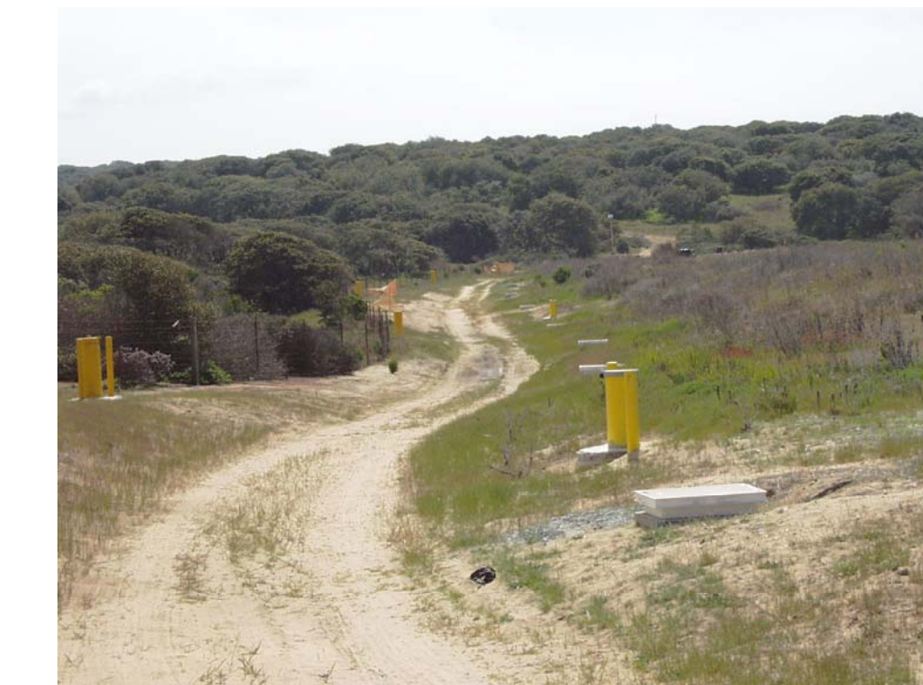
A line of extraction wells at the edge of Area F (to the right in the photograph) extracts landfill gas for treatment. Monitoring probes installed along the fence to the left show that the landfill gas in the soil at the property boundary does not exceed State standards.
