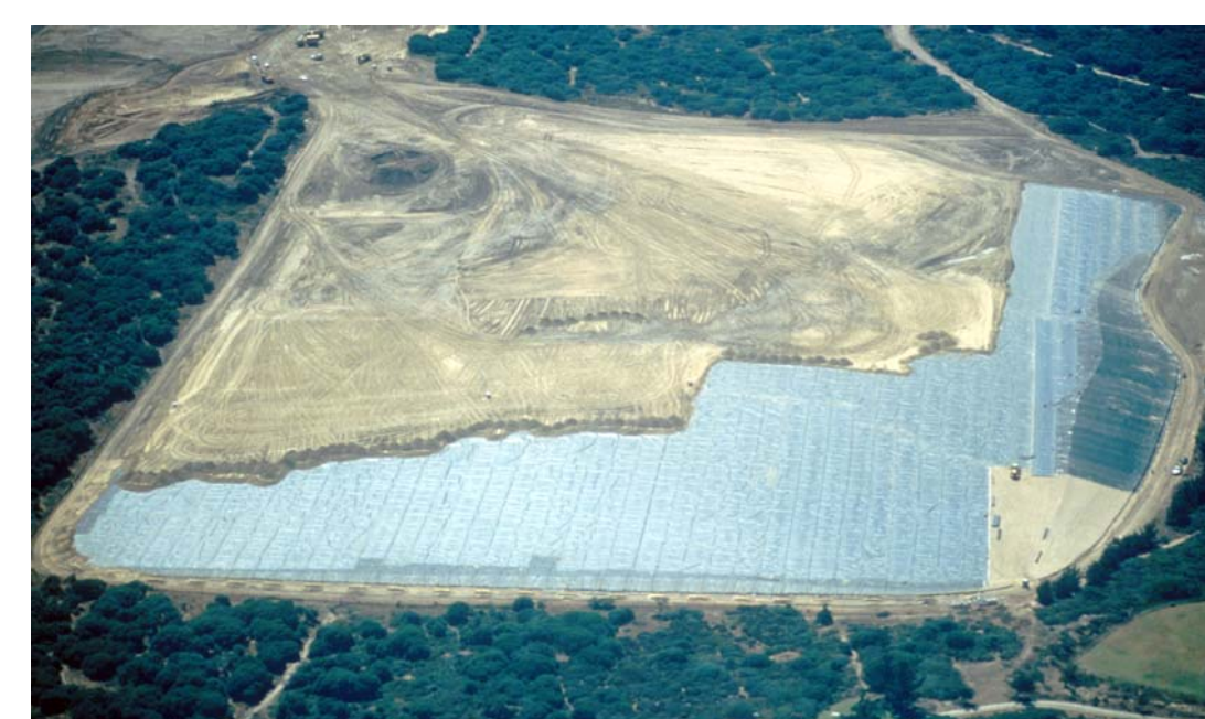
Construction of the engineered cover on Area F in 1998. Clean vegetative cover soil is being spread out over the geomembrane.
