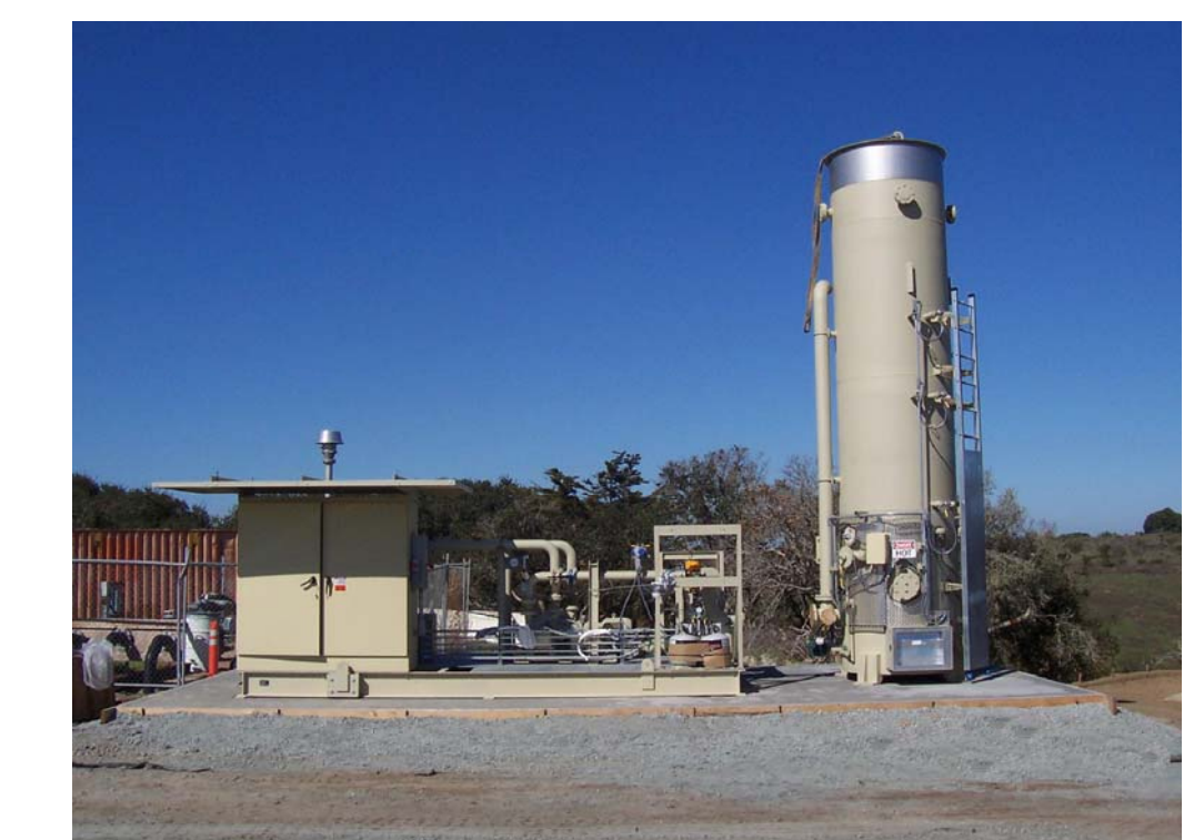
Landfill gas thermal treatment unit installed February 2006.
