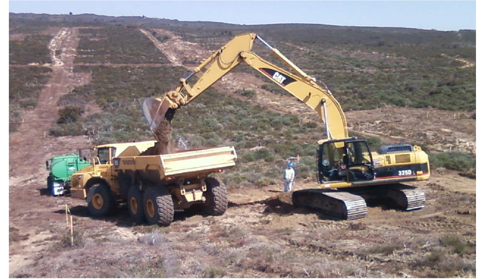
Excavator loads contaminated soil into off-road truck.
